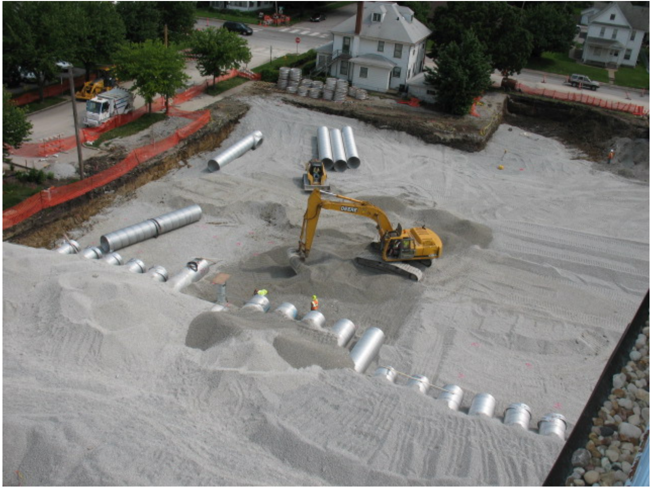
Underground infiltration/detention system under construction.
