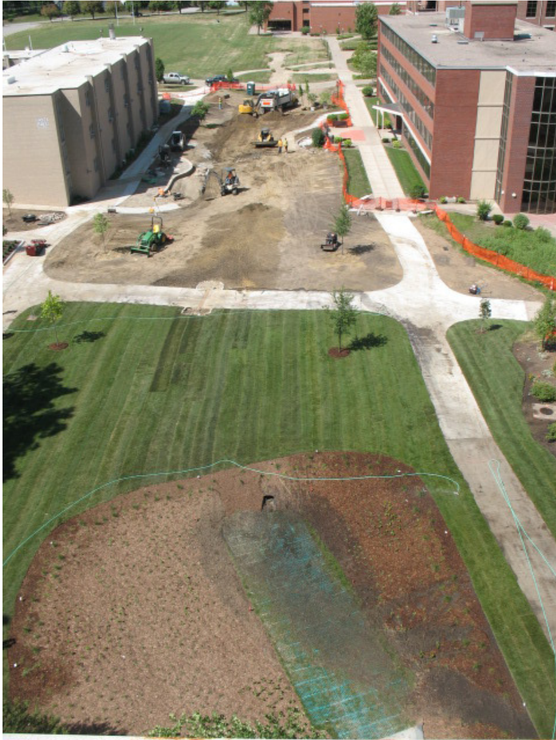
Site grading work in plunge pool/overland flow route area.
