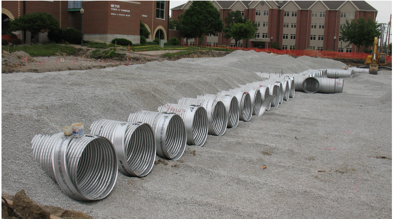
Underground infiltration/detention system under construction.
