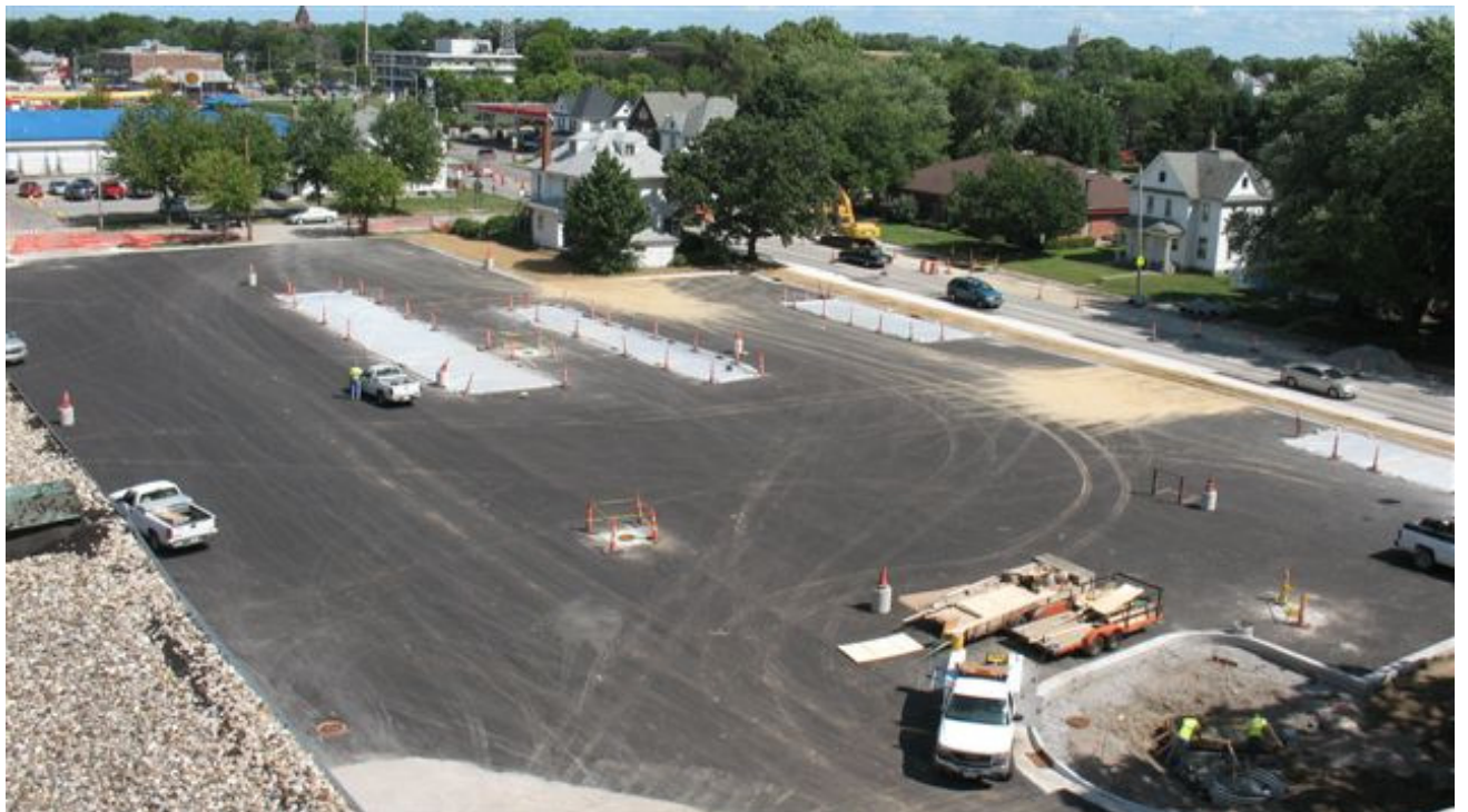
Permeable pavement areas in Cosgrove Parking Lot.
