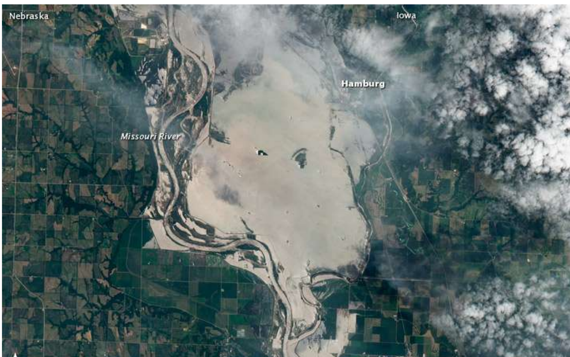
Figure 1: Satellite Image of a Levee Failure near Hamburg, Iowa, Captured on June 24, 2011 (Source: National Aeronautics and Space Administration)
