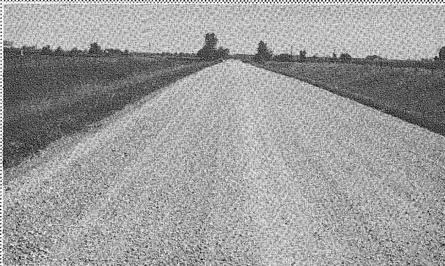
Figure 2 - A road with a high crown. Photo taken in June.
