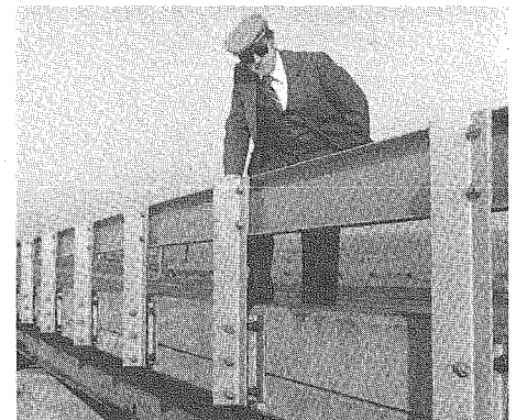
Gene Hales, Pottawattamie county engineer, examines the maintenance-free bridge guard rails and posts that have been dismantled, stripped of old paint and rust, hot-dip galvanized, and reinstalled.
