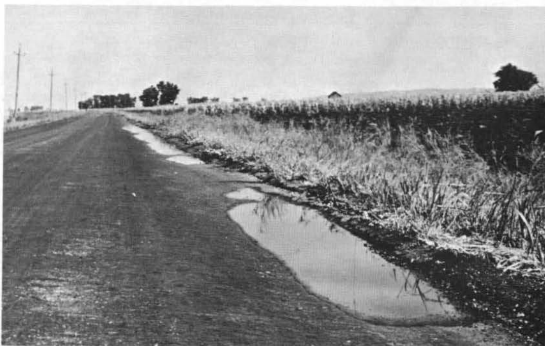
Fig. 15. Cut-back asphalt, in-depth treated surface improvement near De Soto Bend National Park using in-place soil-aggregate. Summer traffic, approximately 4000 vpd. Thickness about 2-2½ in. Age about 1 year.
