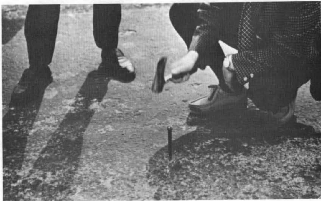
Fig. 12. Lignin-surface treated road. Treatment approximately 2 weeks old.
