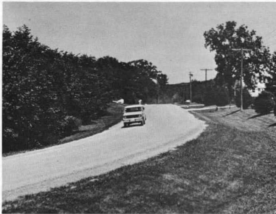
Fig. 13. Lignin plus aluminum sulfate in-depth treated roadway in urban residential area using in-place soil-aggregate. Vehicle speed 40 mph.
