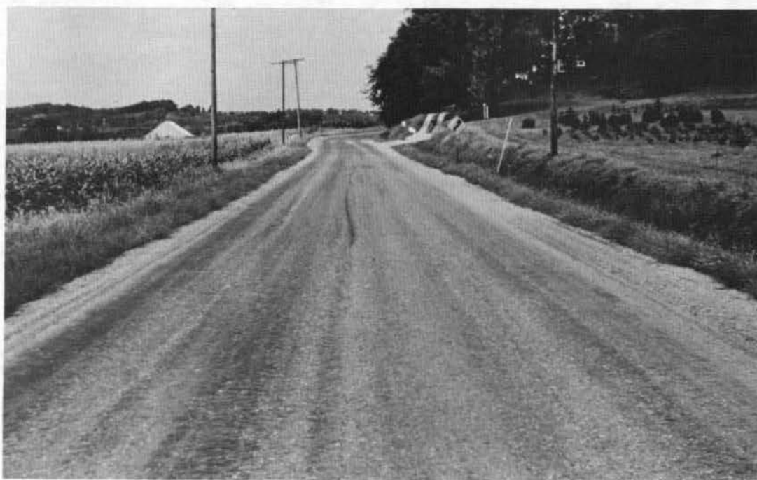
Fig. 16. Cut-back asphalt, in-depth treated surface improvement using in-place soil-aggregate. Traffic, 700 vpd. Thickness about 2-2½ in. Age about 1 year.
