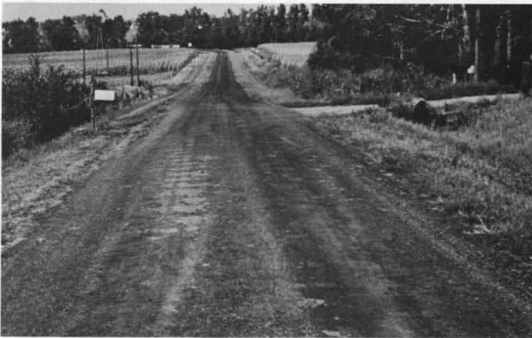
Fig. 10. Oiled road surface showing effects of ravelling and pot holing.
