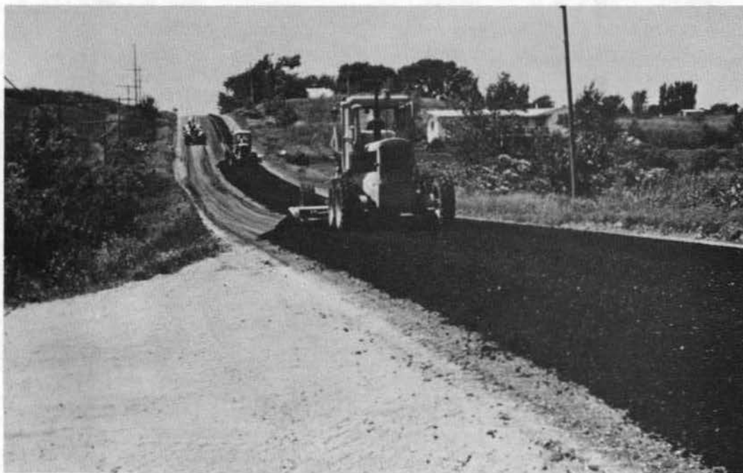
Fig. 14. MC-800 cutback asphalt in-depth treated surface improvement construction using in-place soil-aggregate. Treatment depths about 2-2½ in.
