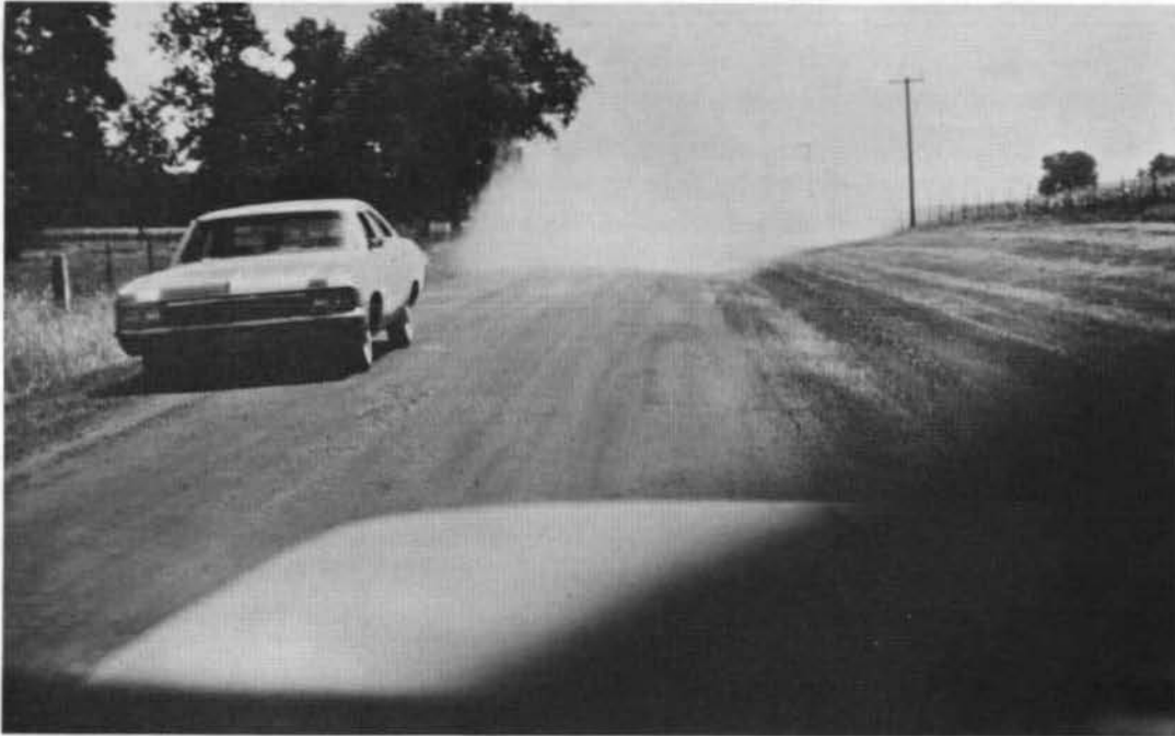
Fig. 9. Oiled road surface in foreground, untreated surface in background.
