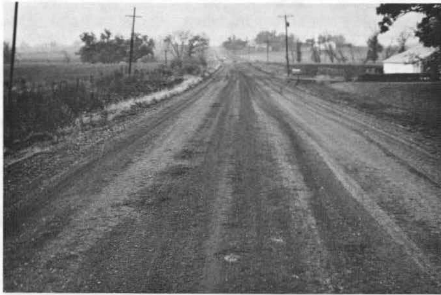
Fig. II-42. Section 5 (2% MC-800) shortly after construction and long drizzling rain, looking west.
