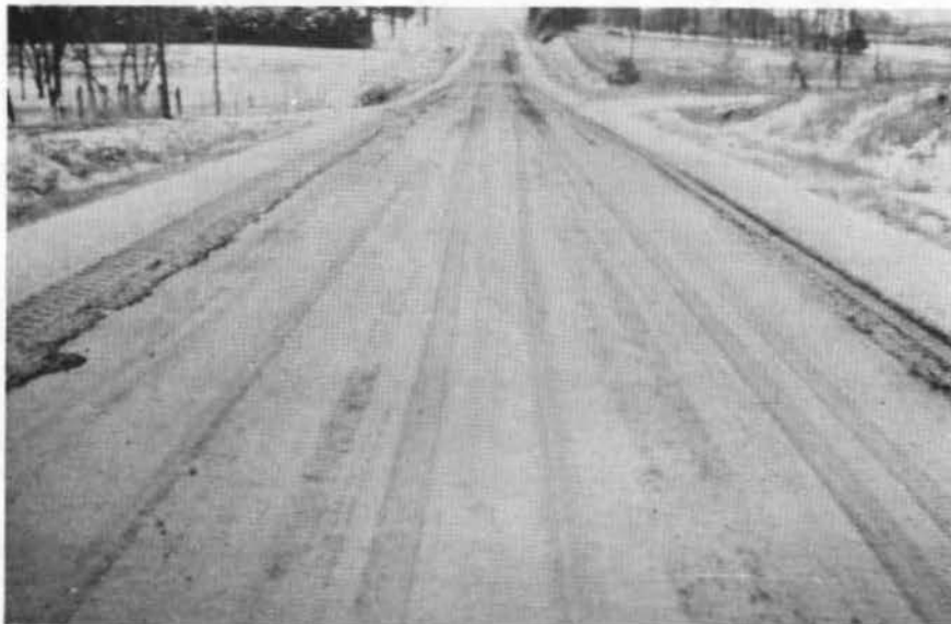
Fig. II-45. Section 8 (4% Redicote emulsion) 3 months after construction, looking east.
