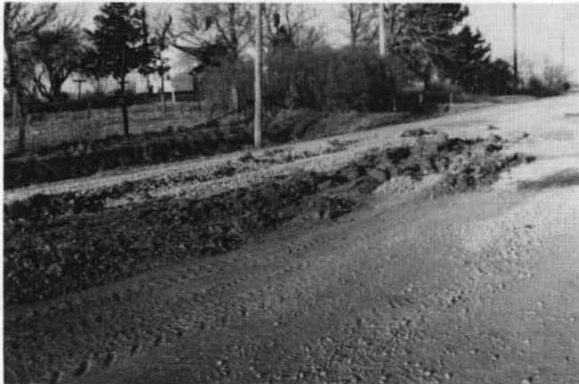
Fig. III-2. Frost boil on unpaved secondary road, Linn County.
