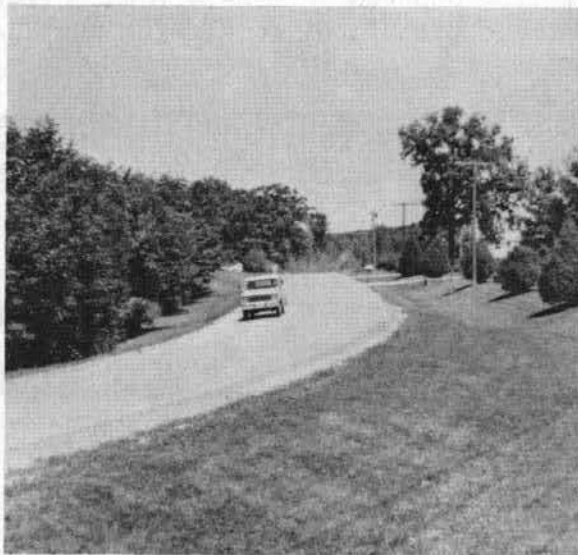
Fig. III-4. Vehicle traveling 40 mph on unpaved secondary road, Linn County, after lignosulfonate in-depth treatment.
