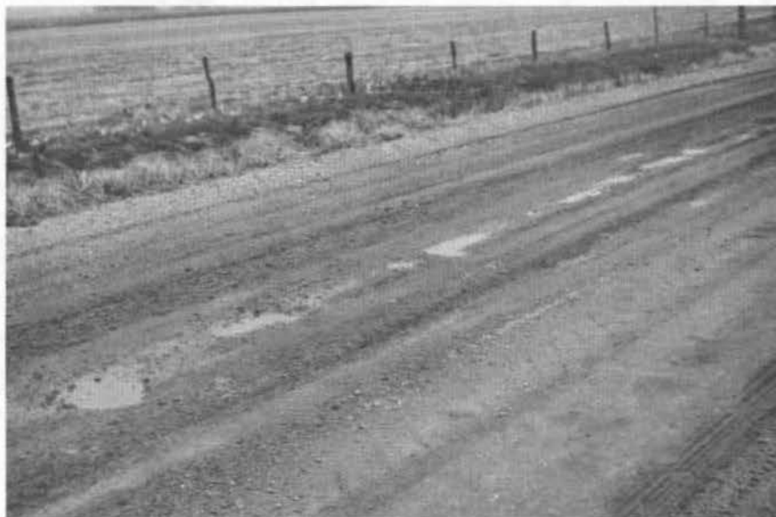
Fig. II-41. Potholing on section 7 (untreated) approximately 1-1/2 months after construction.
