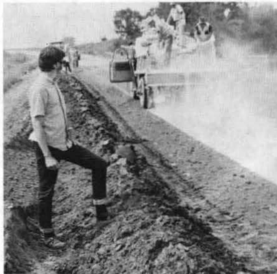
Fig. III-25. Lime spreading during construction, 1970, Clinton test road.
