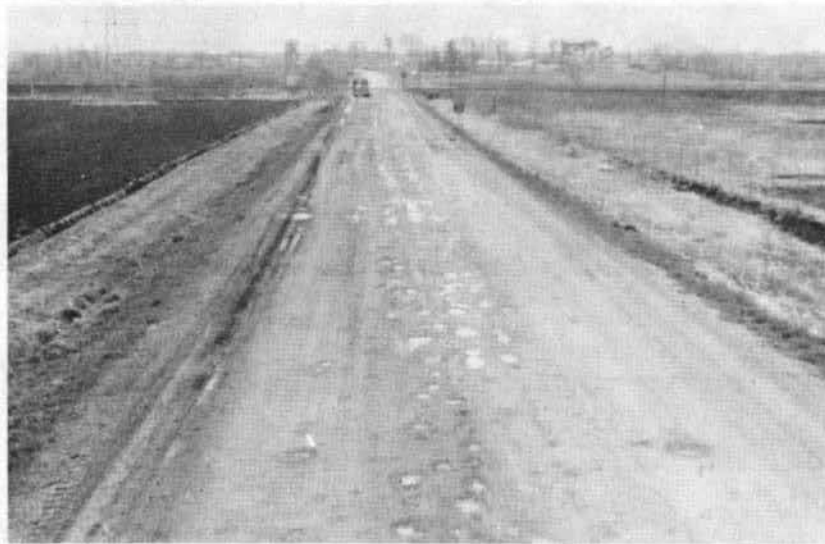
Fig. III-40. 1% lignosulfonate plus 0.5% lime additive section, looking south, spring 1971, Clinton test road.
