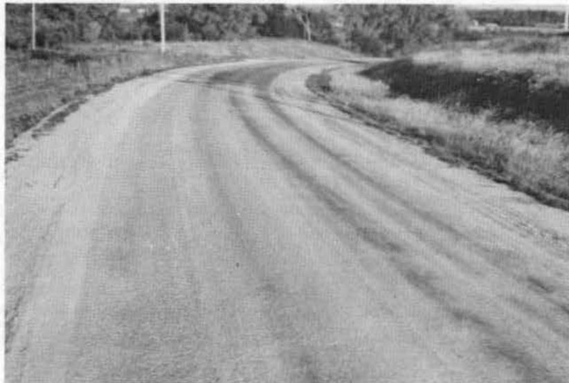
Fig. III-44. Peeling of armor coat during hot weather, fall 1971, Clinton test road.
