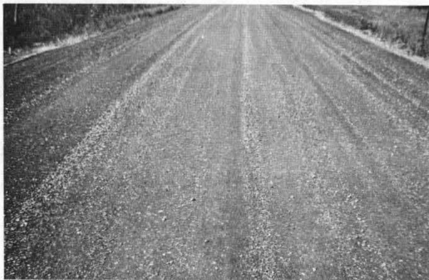
Fig. II-37. Aggregate pullout on section 5 (2% residual asphalt) after construction.
