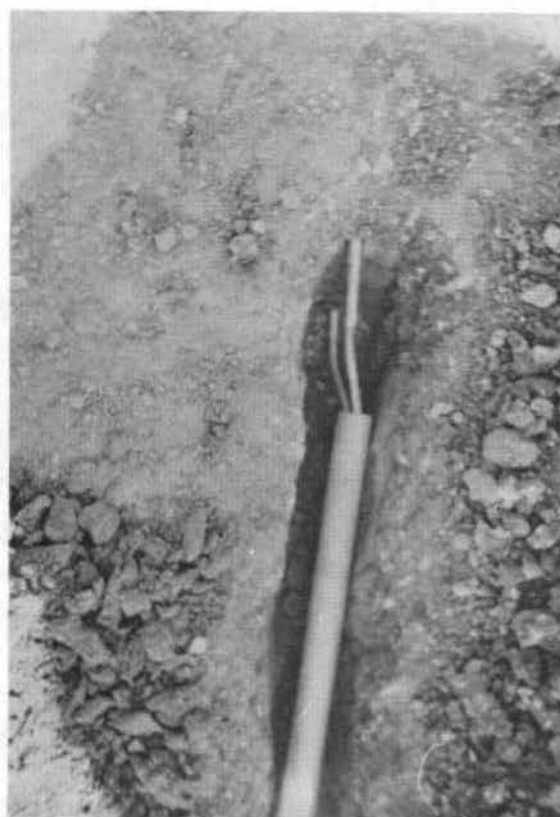
Fig. III-36. Close-up view, dual thermal elements, 1971, Marion test road.
