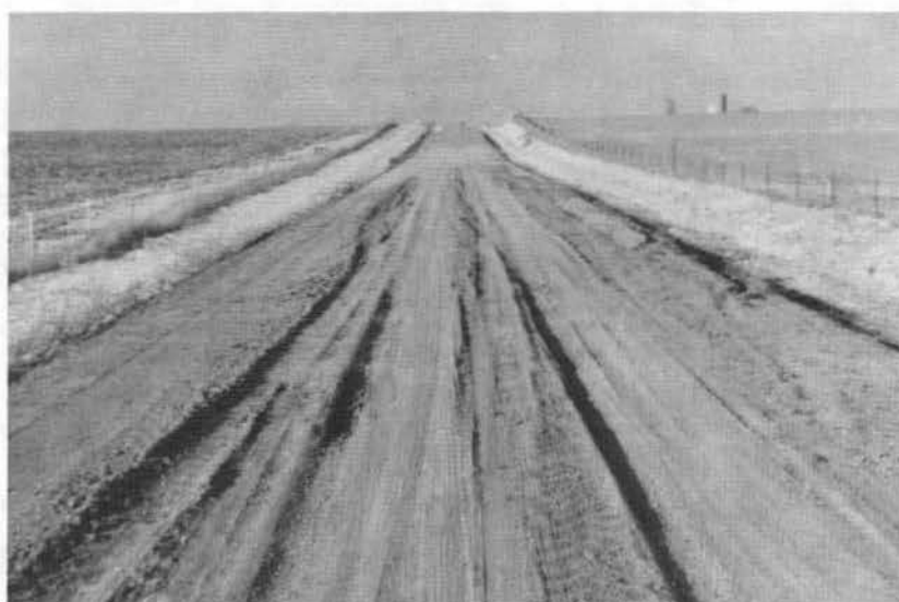
Fig. III-49. Untreated, low aggregate content, section 3, March 1971, Marion test road.
