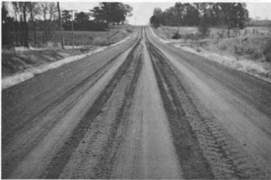
Fig. II-43. Section 8 (4% Redicote emulsion) shortly after construction and long drizzling rain, looking east.
