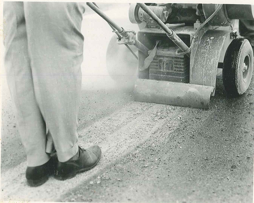
Picture 1 - Close up of G.H. Tennant surface scarifying machine removing bituminous material.
