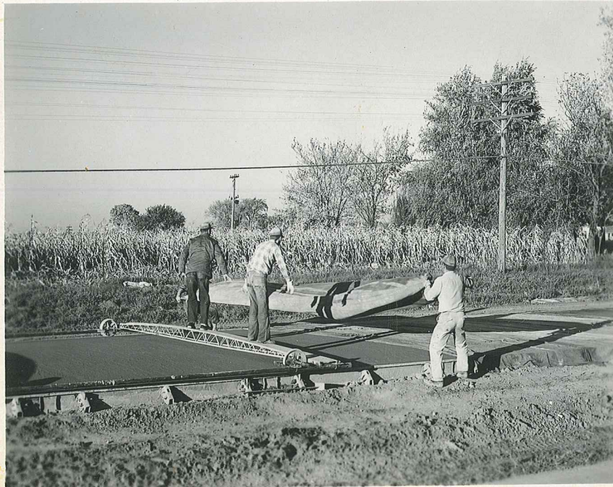
Picture 21 - Initial curing was accomplished with wetted burlap strips.
