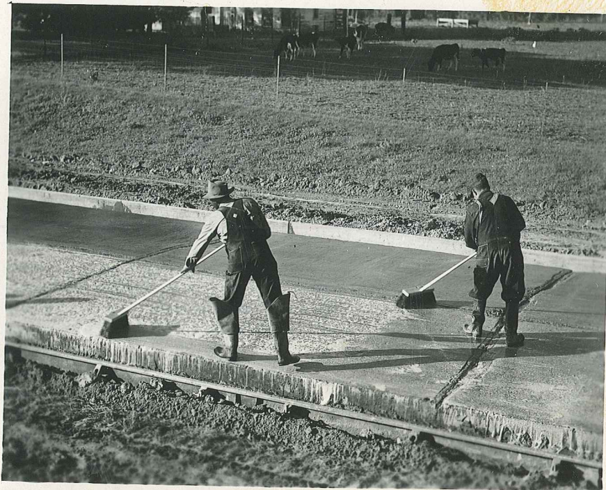
Picture 13 - Acid was further distributed by hand with rattan brooms.
