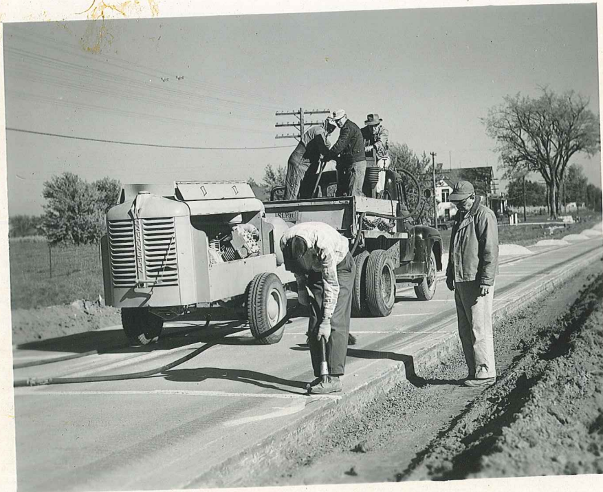
Picture 3 - Sand blasting bituminous material from routed out joints and cracks.
