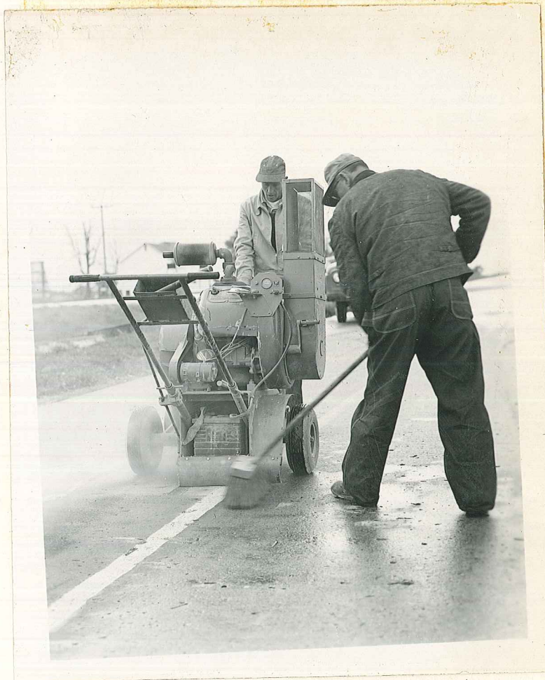
Picture 2 - Removing center line paint stripe from old pavement surface.
