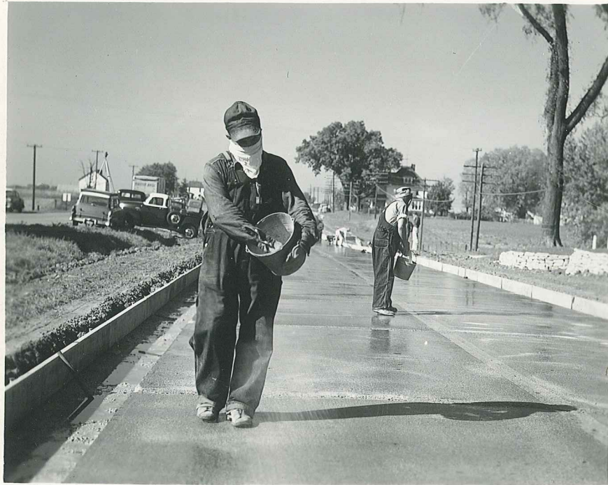
Picture 9 - Metzo 66 detergent was spread by hand at rate of 2 lb. per 100 sq. ft.
