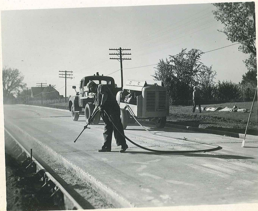
Picture 7 - Loose material being blown from crack crevices with air jet.
