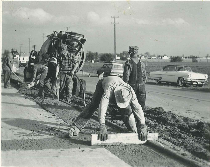
Picture 17 - Concrete for widening was placed from transit mixers, vibrated into place and struck to grade by hand.
