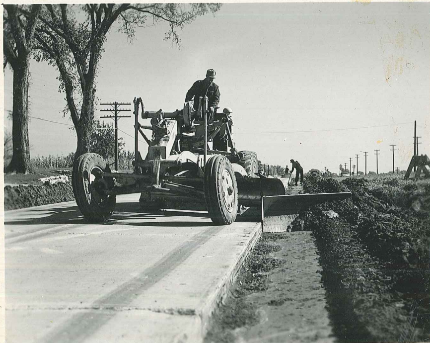
Picture 4 - Excavating trench, for widening using blade grader with trenching attachment.
