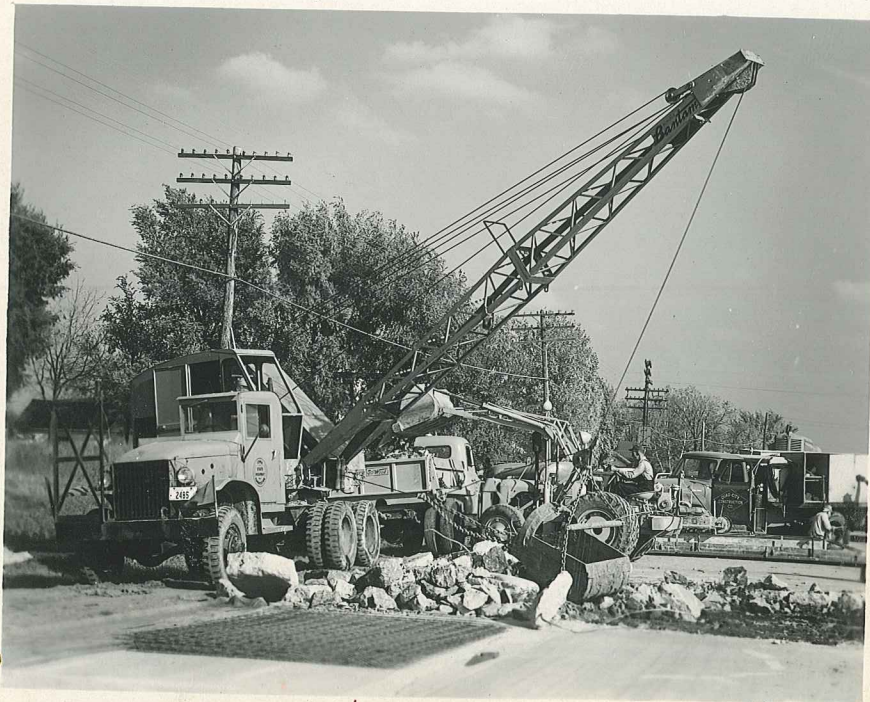
Picture 15 - Concrete being removed for 32 foot ramps placed at both ends of project.
