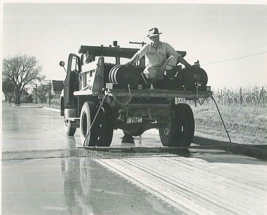
Picture 11 - Detergent residue was flushed from pavement until it showed neutral with pH paper. Same equipment used to flush surface after etching with acid.
