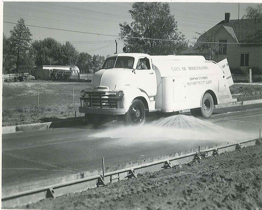
Picture 11 - Detergent residue was flushed from pavement until it showed neutral with pH paper. Same equipment used to flush surface after etching with acid.
