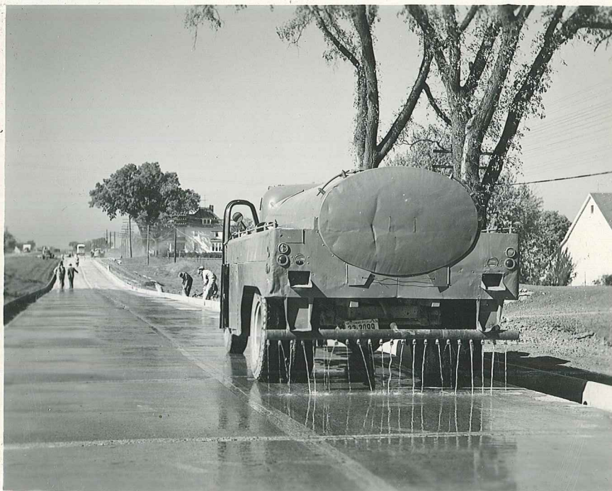
Picture 8 - Old pavement surface being wetted by tank truck equipped with spray bar. Surface was sprinkled ahead of applying detergent and acid.
