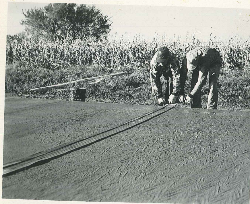
Picture 20 - Final surface finish was by hand operated transverse belt.
