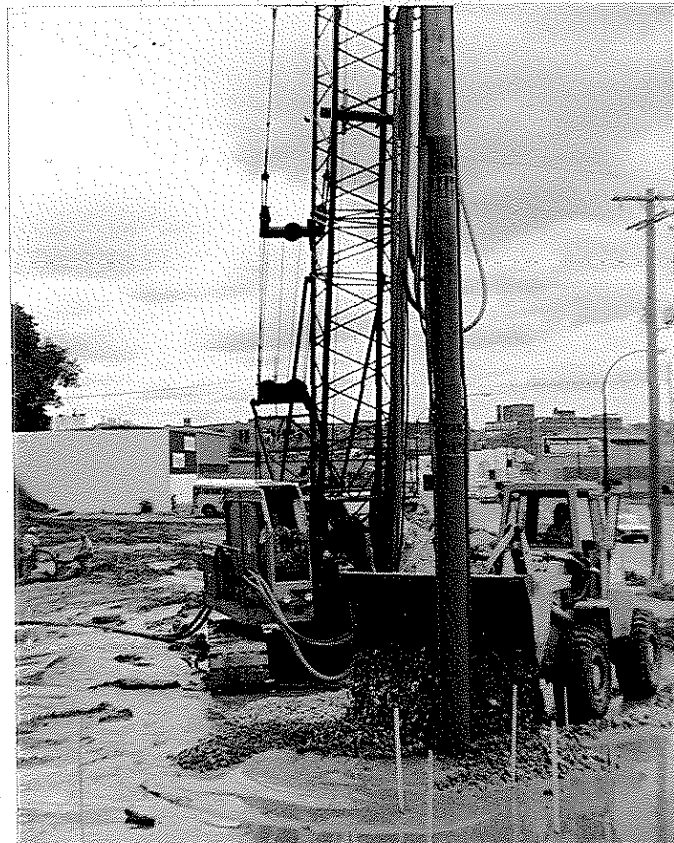
Stone Column Installation
