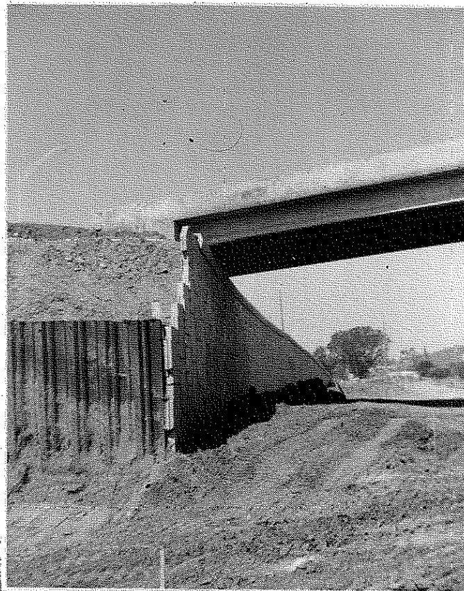
Stage Construction-Reinforced Earth Wall No. 3
