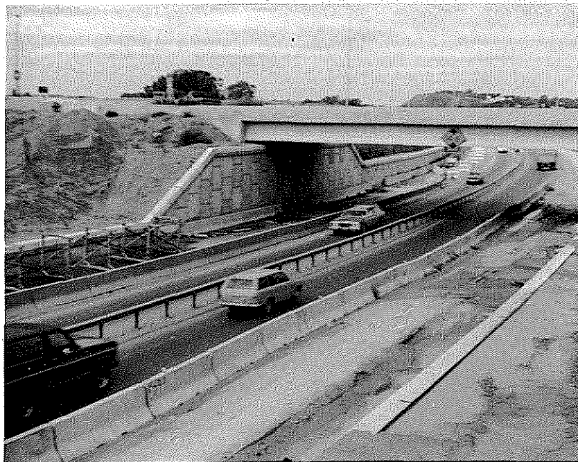
Completed Reinforced Earth Wall No. 1 (Top of Wall 2 is in foreground)
