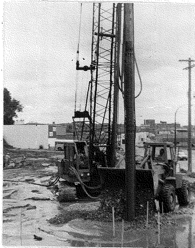
Stone Column Installation
