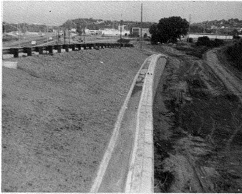
Wall distortion-Reinforced Earth Wall No. 3 West End (Page 4 and 5)
