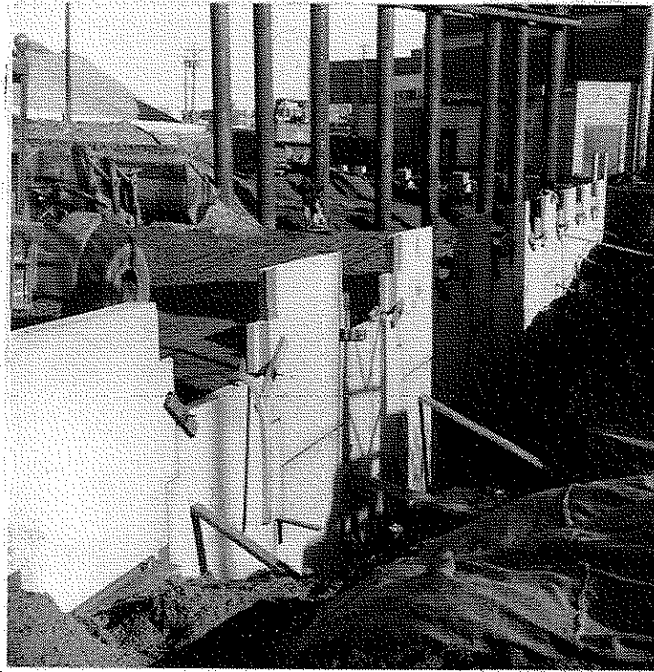
Beginning of construction-Reinforced Earth Wall No. 4 Pile covering can be seen (Page 4)
