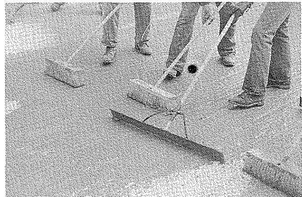
Applying Grout
