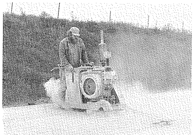
Sawing Transverse Joint
