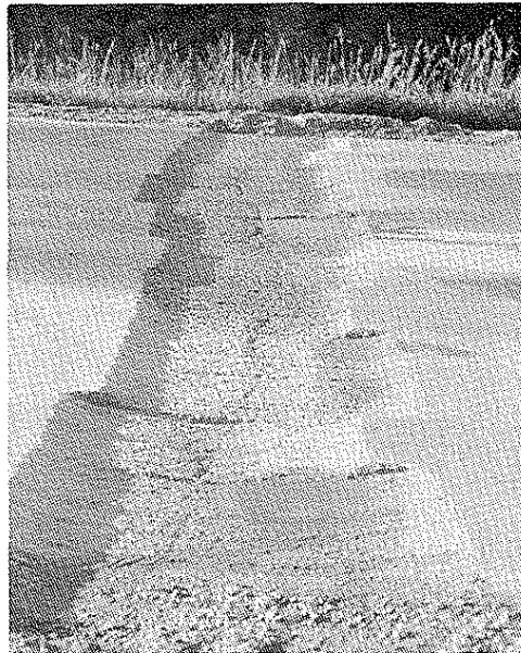
Partial Depth Joint Scarification
