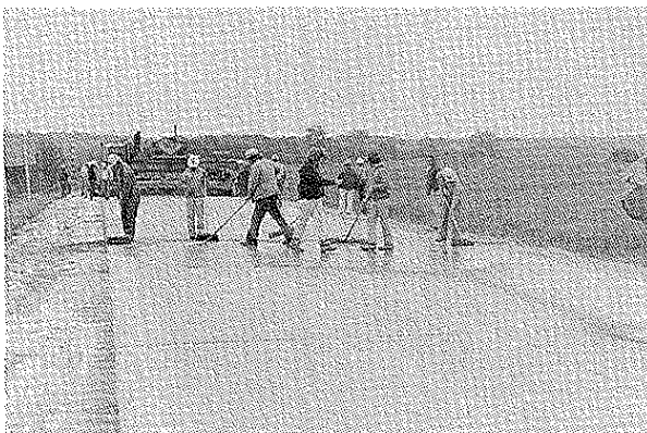
Applying Grout
