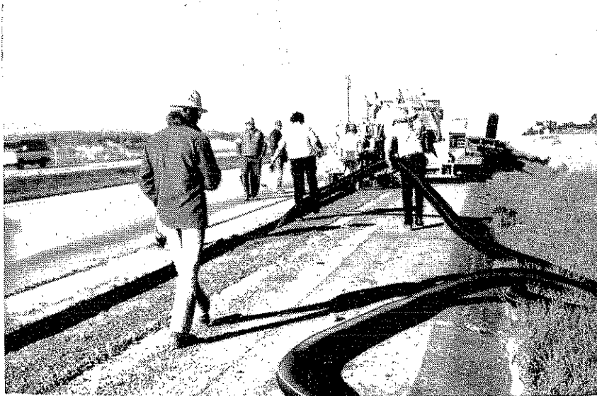
Figure 4: Hand Placement of the Tubing
