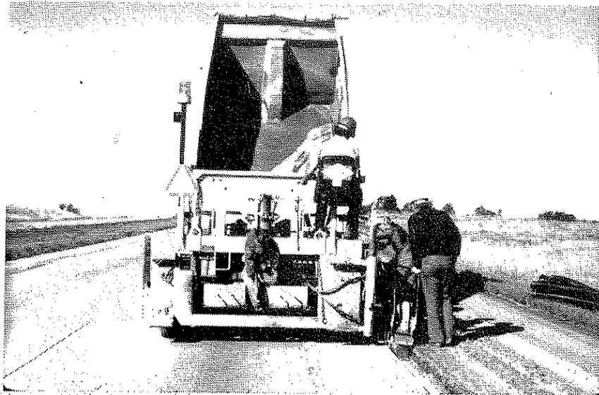
Figure 5: Blawnox RW-38 Placing Porous Backfill
