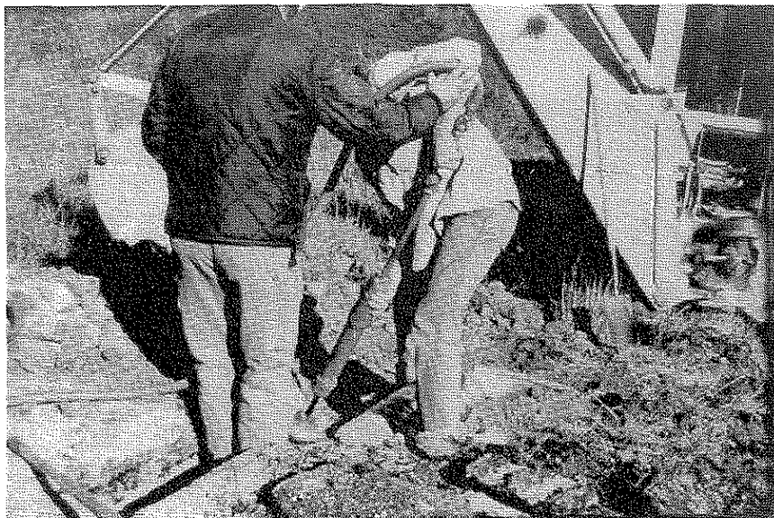
Figure 10: Tamping Earth Fill Around the RF-22 Outlets
