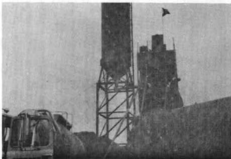
FLY ASH SILO IN PLACE
