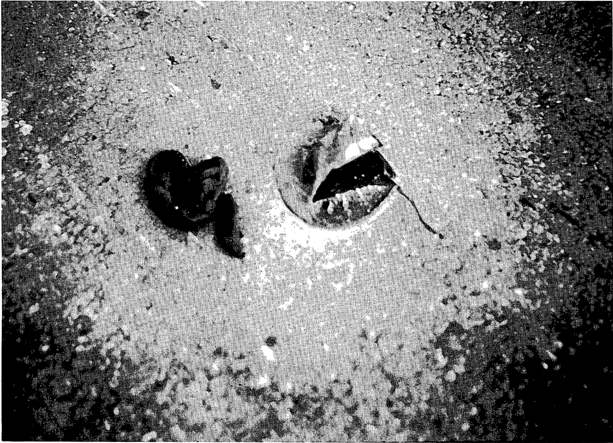
Figure 6 - Sealant Material Tracked by Traffic
