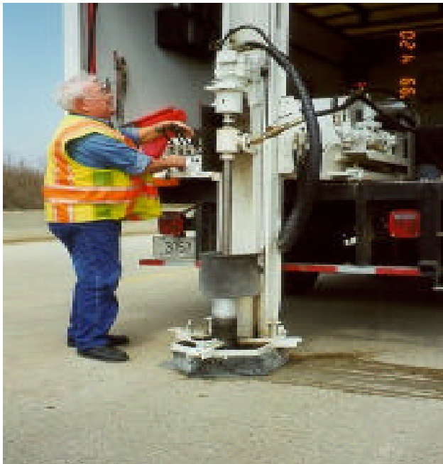
FIGURE 4.2 The Setup of the Coring Process
