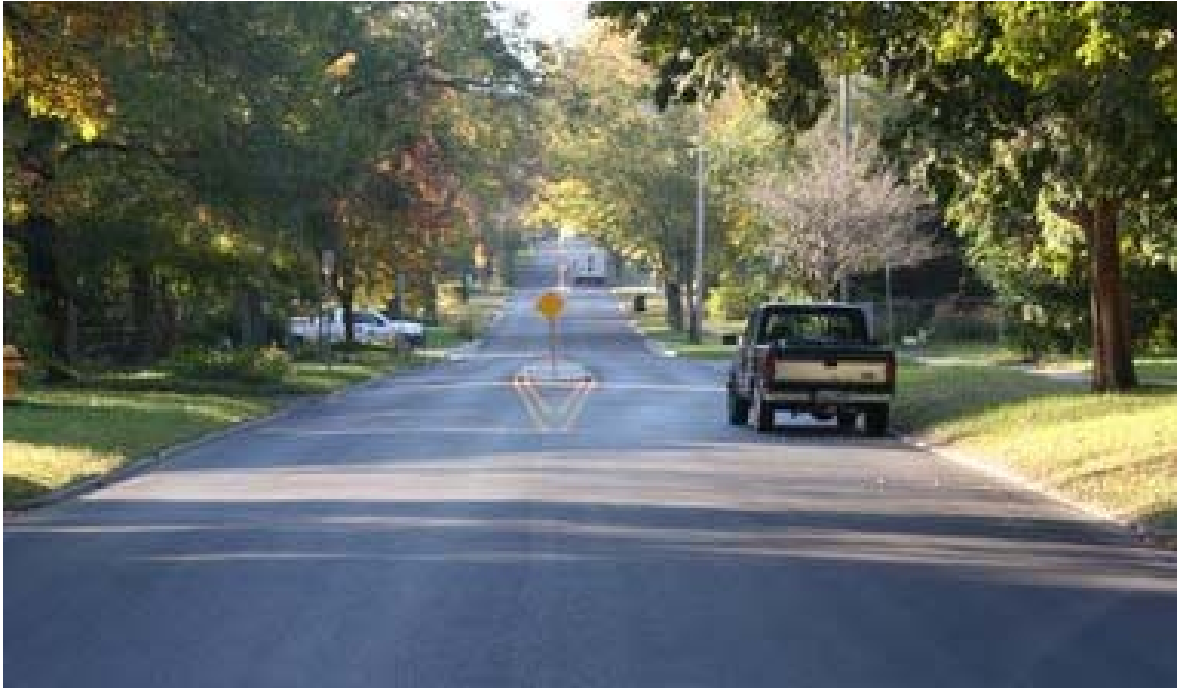
Figure 3.12. Use of a small, painted center island (source: Isebrands)
