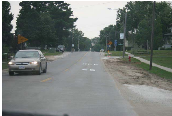
Figure 5.20. On-pavement speed signing
