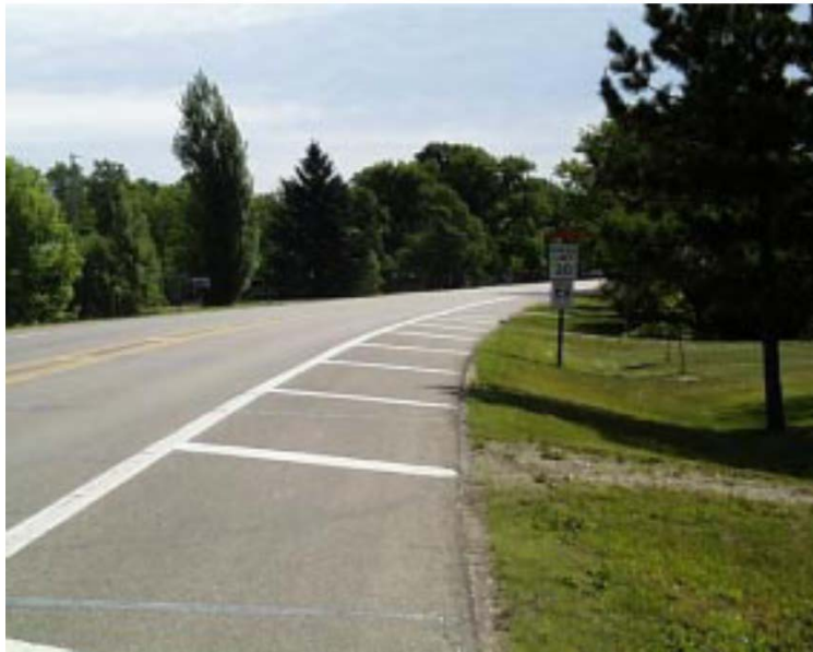
Figure 3.35. Lane narrowing with transverse shoulder stripes
