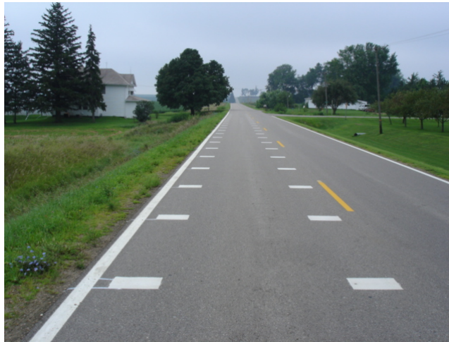
Figure 3.22. Optical speed bars used in Union (facing back towards markings)
