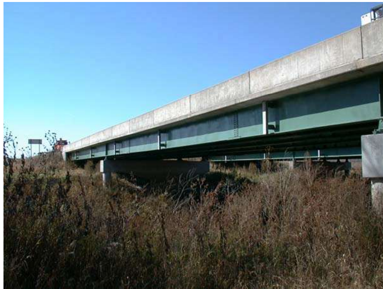
Figure 2.1. Photograph of test bridge looking northwest.
