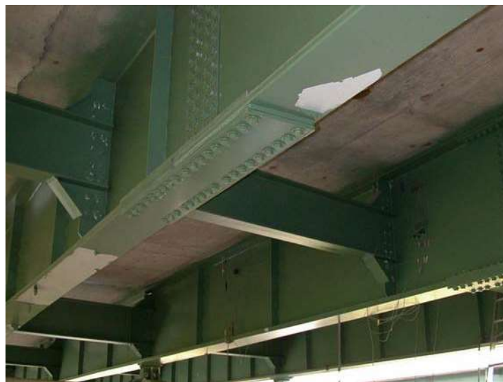
Figure 2.5. Photograph of underside of the bridge looking northwest.
