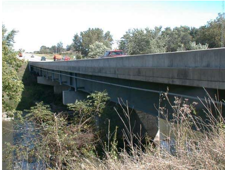
Figure 4.1. Photograph of bridge looking northeast.
