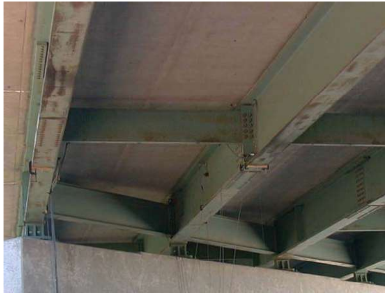
Figure 3.5. Underside view of diaphragm and girders.
