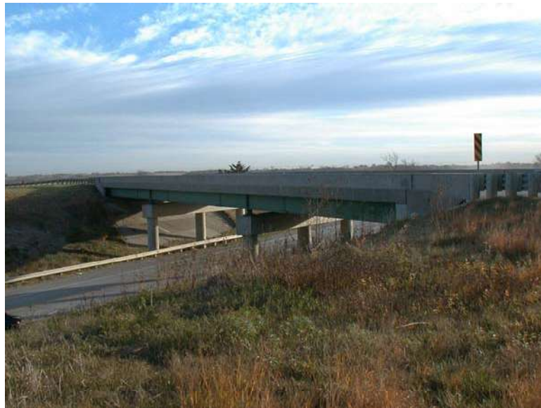
Figure 3.1. Photograph of test bridge looking northeast.
