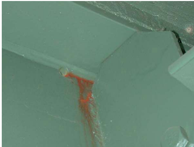
Figure 2.11. Photograph of typical drilled hole retrofit in a web.
