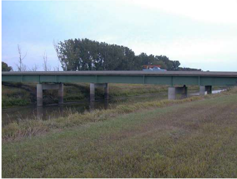
a. Photograph of bridge looking northeast.
