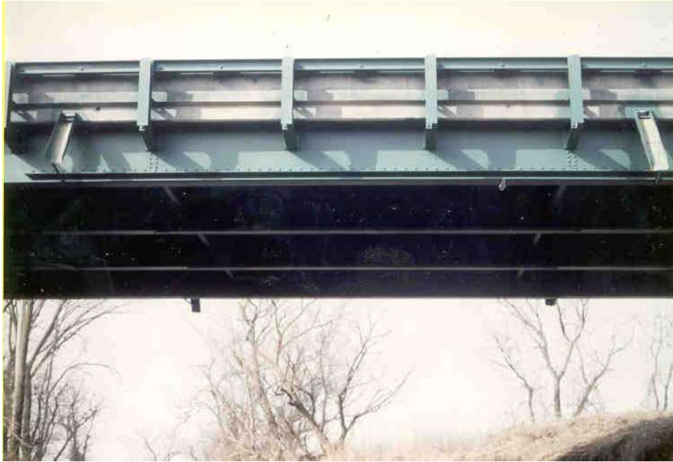
(a) Exterior Girder Strengthened Using Angle Stiffeners
