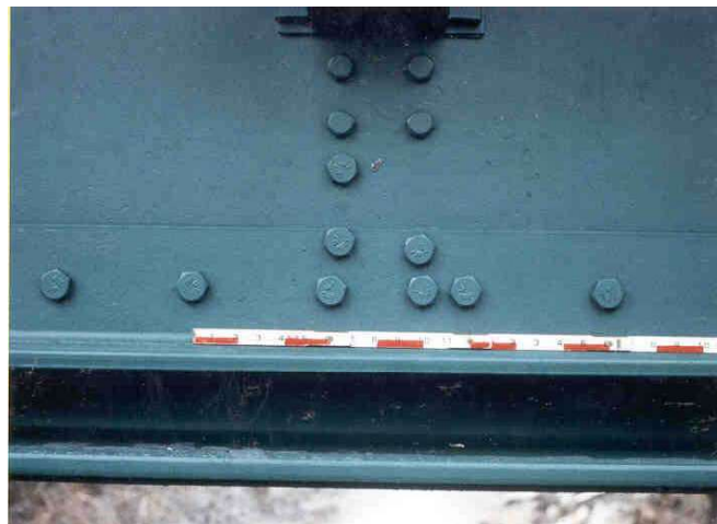
(b) Close up View of the Angle Stiffeners
