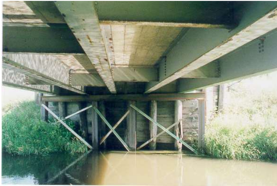
(b) Strengthening by Addition of Supplementary Steel Piles
