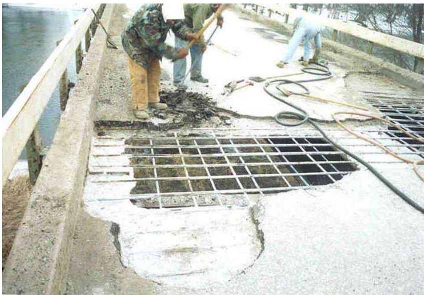
Figure 2.3.16 Full Depth Deck Patching.
