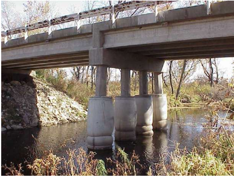
(a) Jacketing of Concrete Piles
