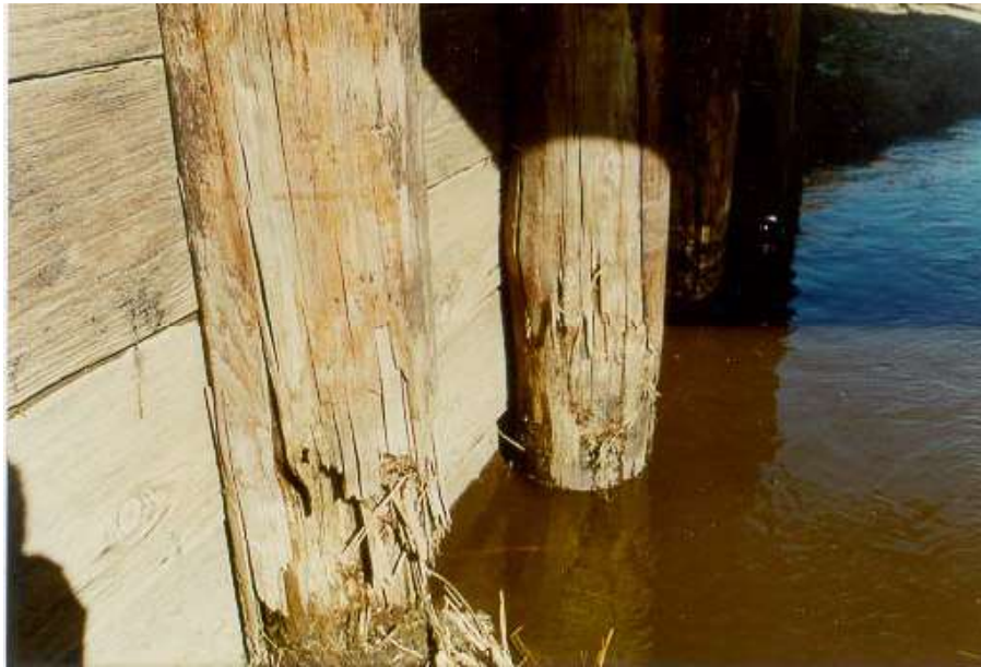
(a) Deteriorated Pile
