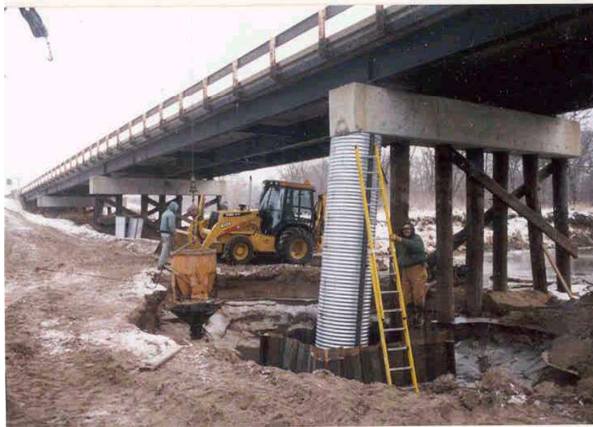
(b) Jacketing of Timber Piles
