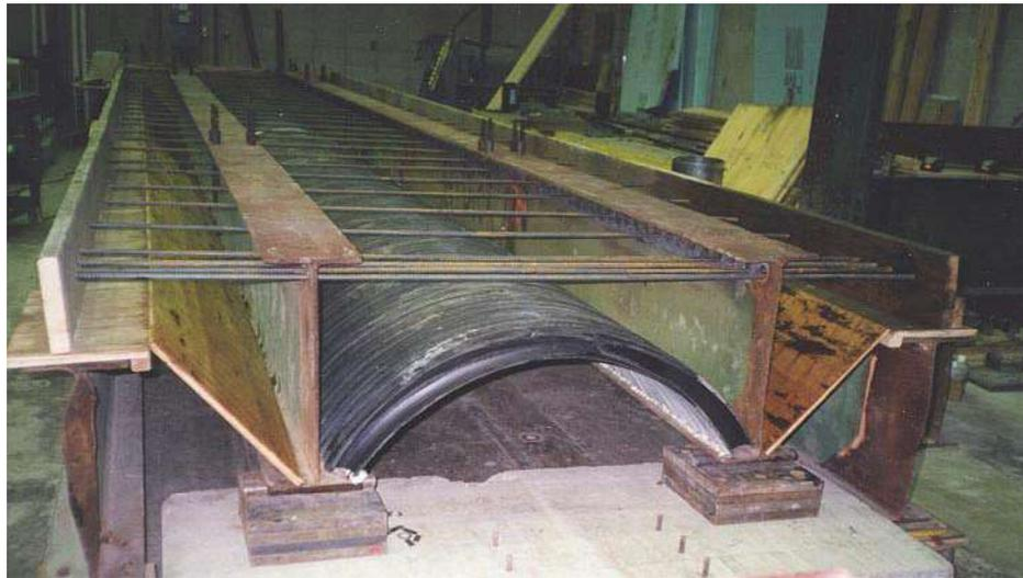
c. Photograph of formwork and reinforcement
