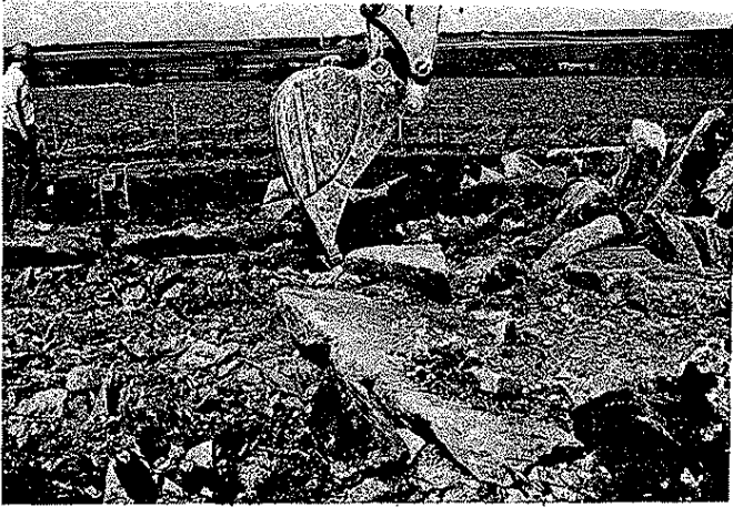
Figure 3 Removing Broken Concrete
