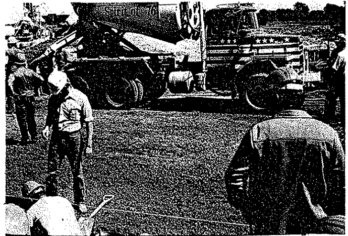
Figure 8 Harsh Concrete in Lower Course of Composite Section
