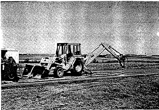
Figure 1 Punching Holes in Old Pavement
