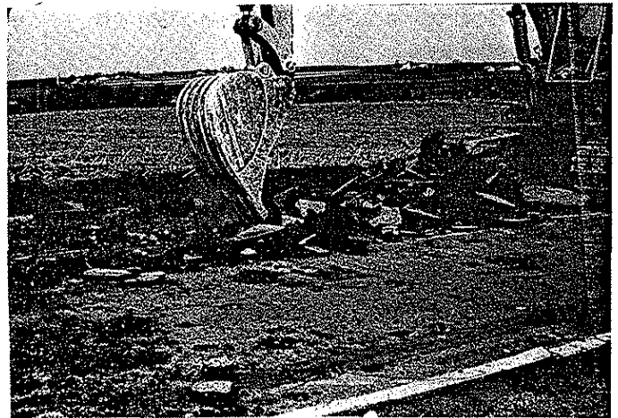
Figure 2 Removing 3 in. A.C. Resurfacing
