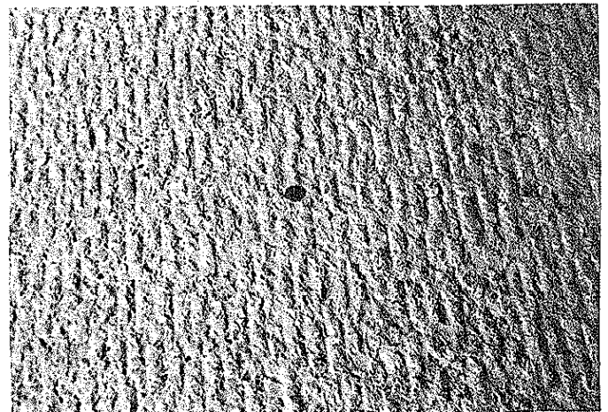
Figure 6 Scarified surface
