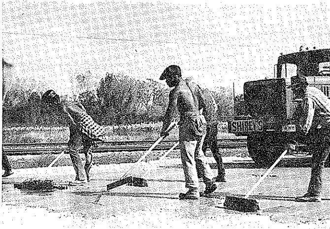
Figure 7 Workmen Spreading Grout
