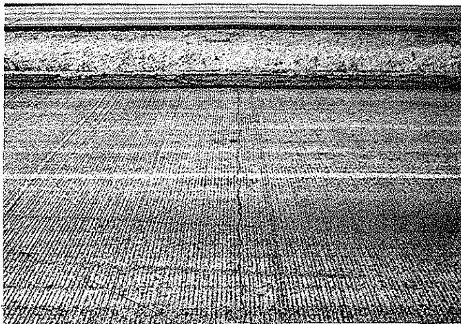
Figure 14 Reflected Transverse Crack in Resurfacing
