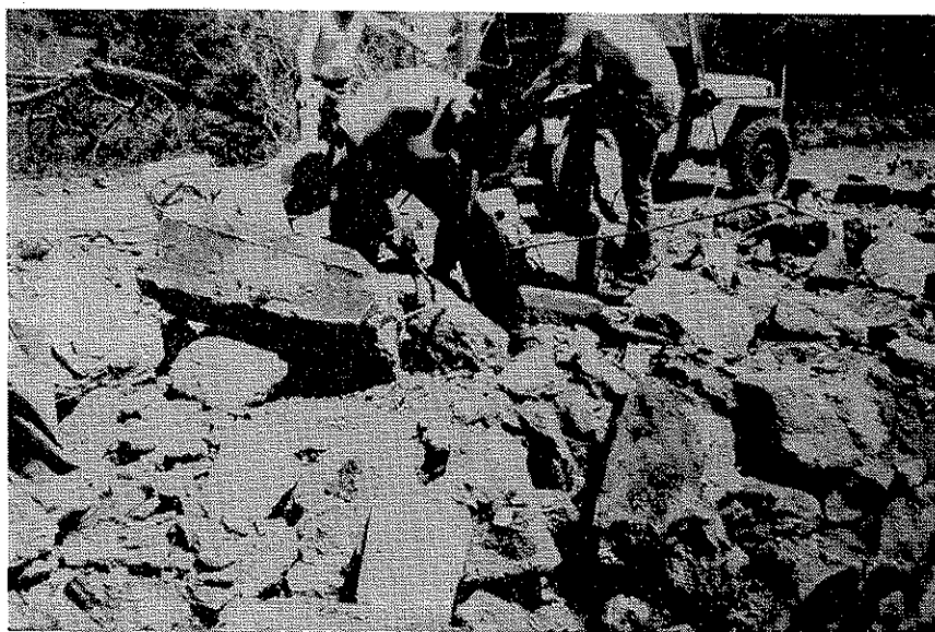
Figure 8: Removing the steel with a cutting torch
