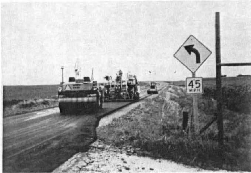
Photo 7: Paving and Rolling Equipment
