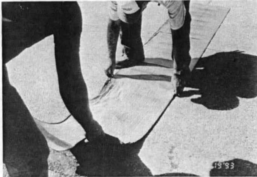
Photo 1: Placement of PavePrep
