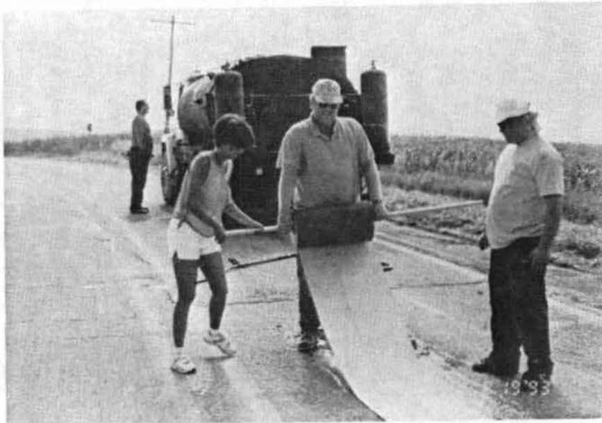
Photo 2: Placement of Pro-Guard
