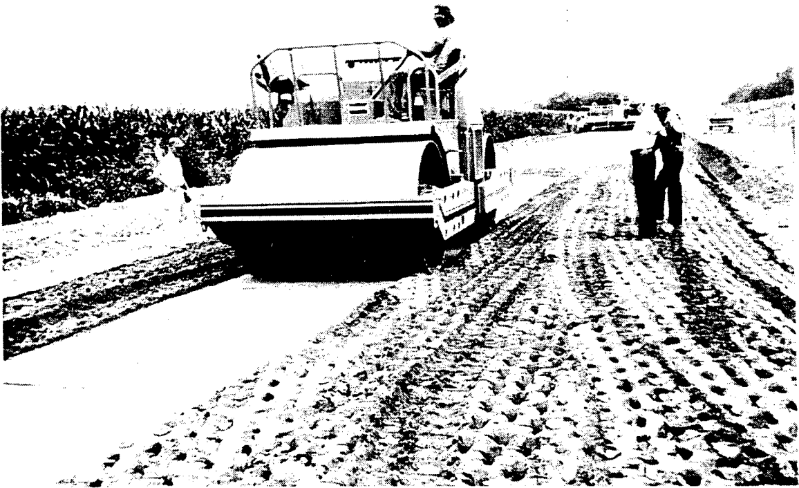
Figure 7 Double Drum Roller Performing Final Consolidation
