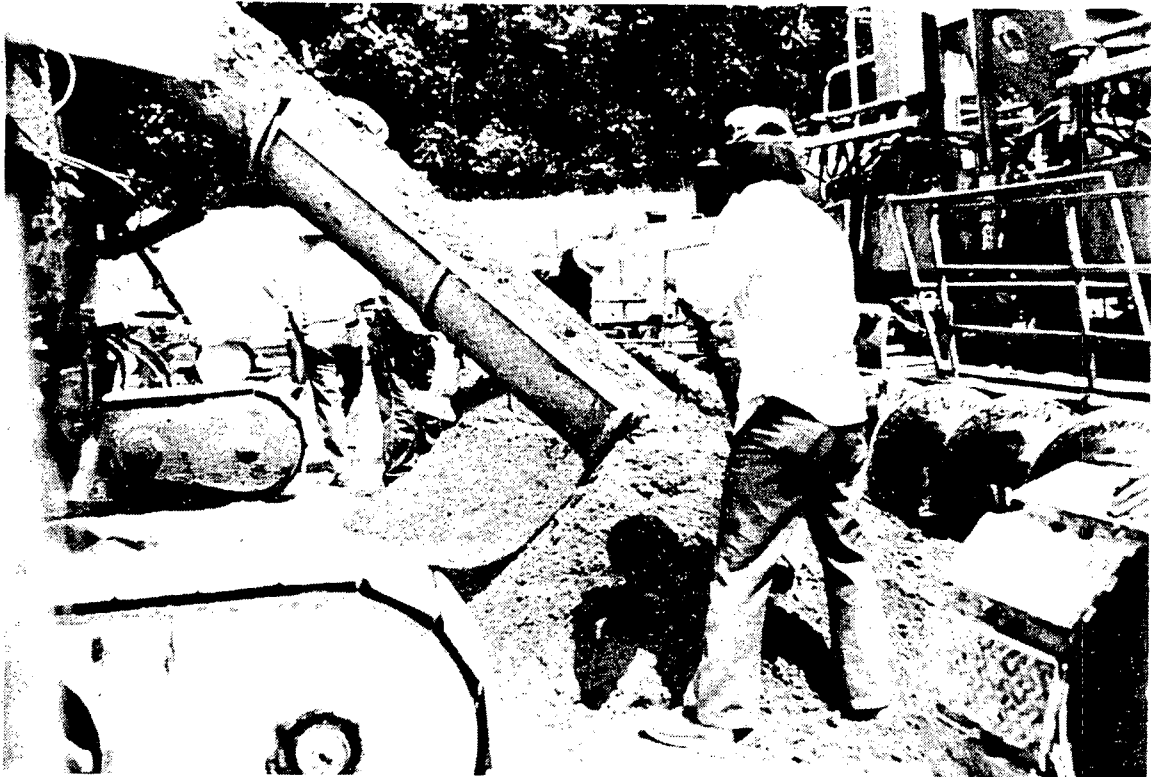
Figure 5 Subgrader Depositing Mix Ahead of Paver
