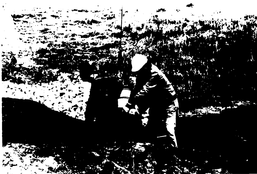
Photo 14 Threading "Culvert Renew" Liner Segment by Hand (Taylor County)
