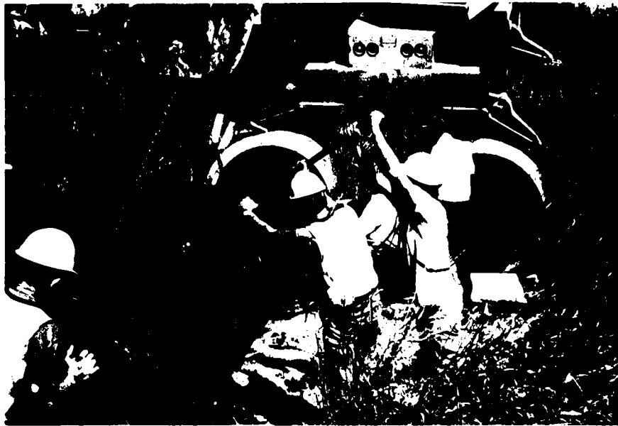
Photo 5 Threading "Culvert Renew" Liner Segments in Jones County
