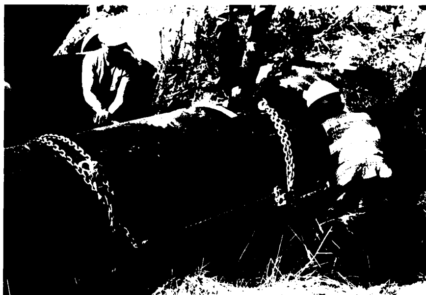
Photo 8 Connecting "Snap-Tite" Liner Segments (Jones County)
