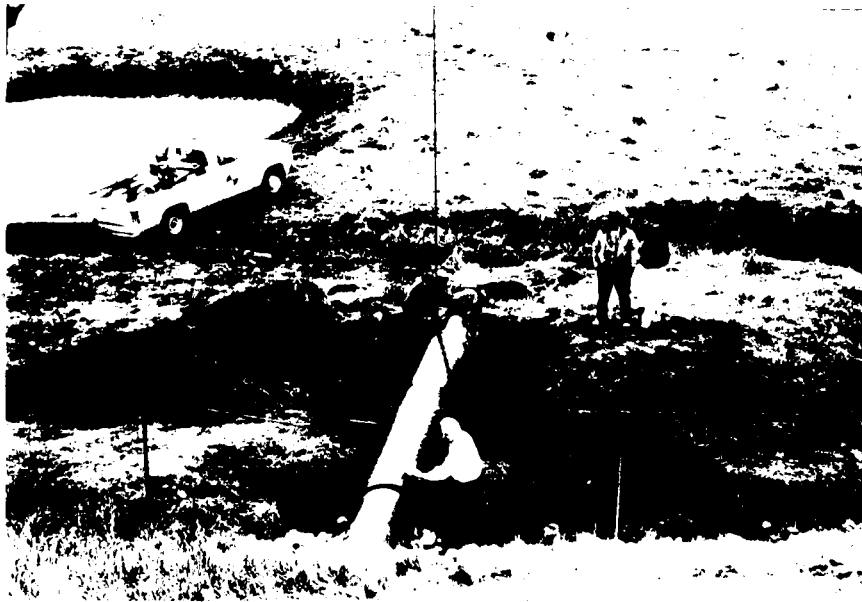
Photo 15 Work Area for Assembling Liner (Taylor County)
