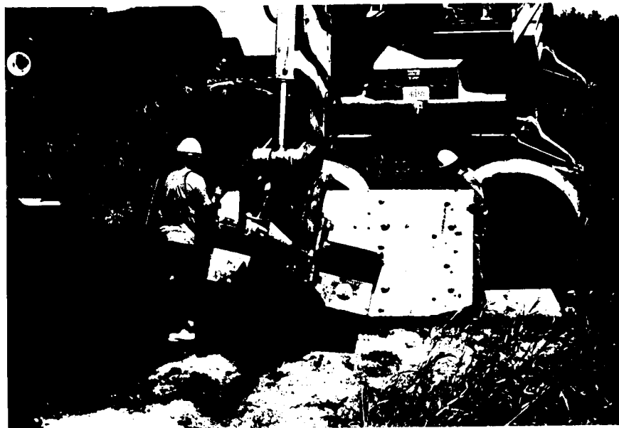
Photo 6 Use of a Board to Protect the Culvert Liner While it is Pushed into the Concrete Culvert (Jones County)
