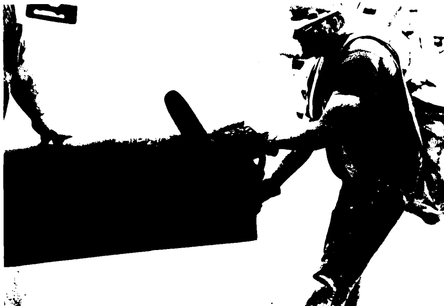
Photo 16 Cutting of Nose Cone With Chain Saw (Audubon County)
