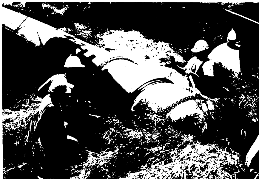
Photo 7 Connecting "Snap-Tite" Liner Segments (Jones County)
