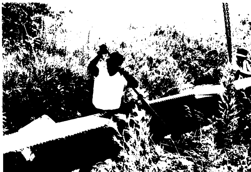
Photo 11 Threading "Culvert Renew" Liner Segments (Mahaska County)
