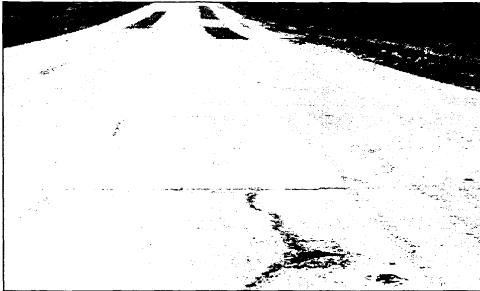
Figure 5 - Full depth and surface patches on a patch only section
