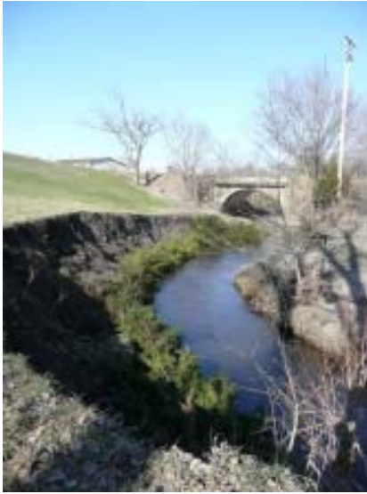
Figure 1. Looking downstream. Red cedar revetment is on the left side of the stream. Picture taken April 14, 2009.
