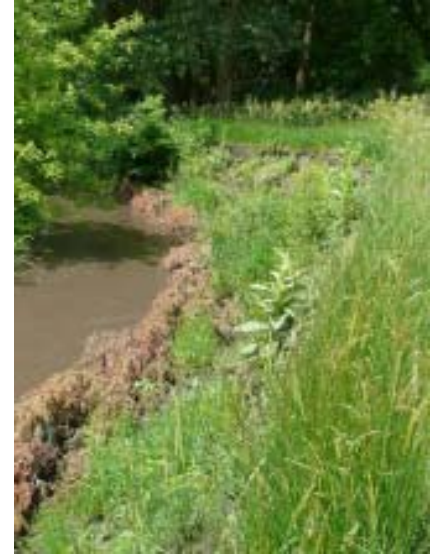
Figure 3. Looking upstream. Red cedar revetment is on the right side of the stream. Picture taken June 19, 2009. Note vegetation regrowth to the right of the revetment along the bank is hiding the willow cuttings from Figure 2.
