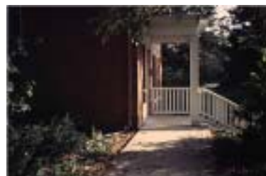
Figure 2: Side view of home entrance with section of porch railing removed. A gently sloping sidewalk creates a no-step design that is integrated with porch and surrounding landscape.
