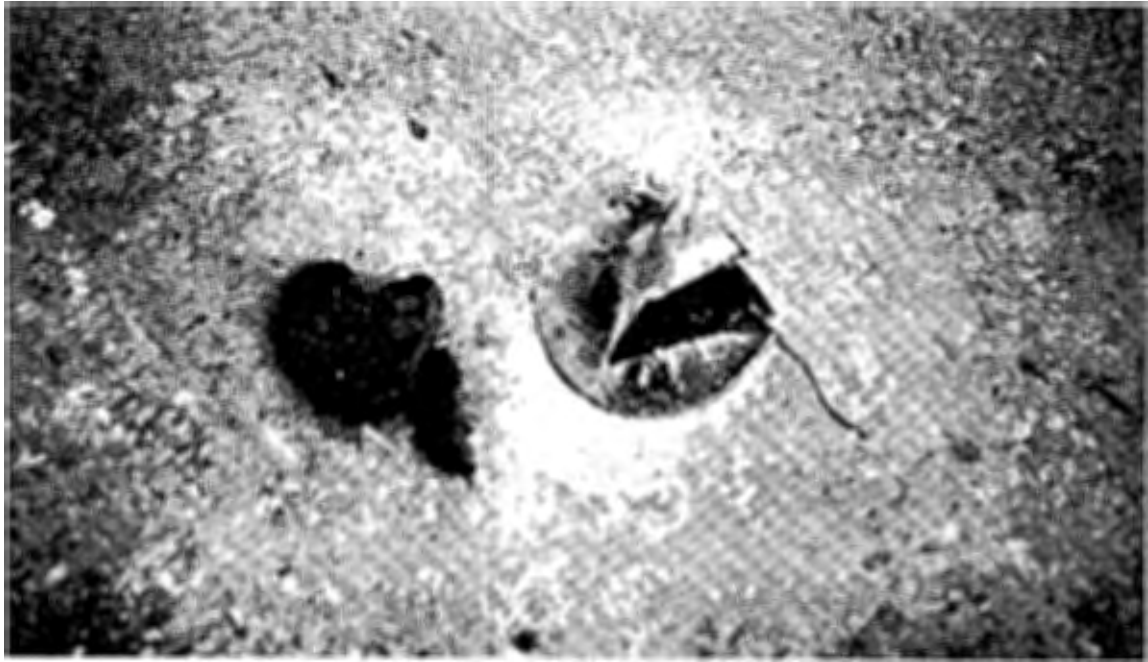
Figure 8 - Sealant Material Tracked by Traffic
