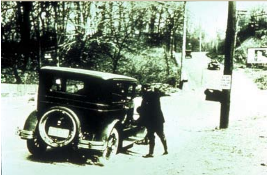
A horn-actuated traffic signal. The microphone is the black box hanging on the pole on the right.
