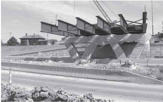
Current bridge construction on I-235 in Des Moines
