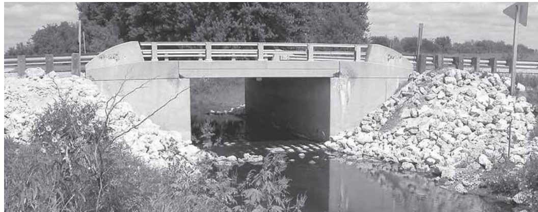
(photo below) Flooding caused scour to occur around the abutments of the U.S. 18 bridge in Chickasaw County. (photo above) After the flood waters receded, repairs were made and countermeasures installed intended to help prevent future scouring.
