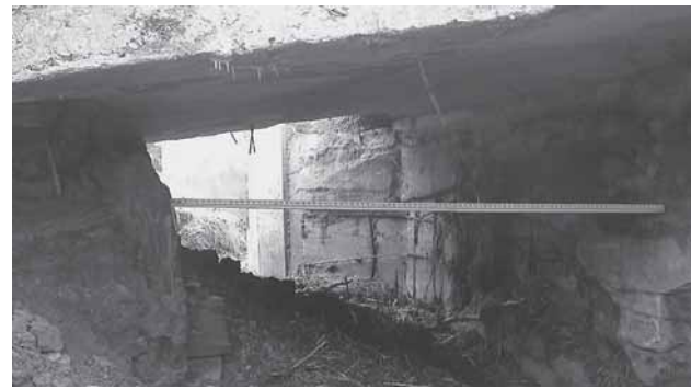
(photo below) Flooding caused scour to occur around the abutments of the U.S. 18 bridge in Chickasaw County. (photo above) After the flood waters receded, repairs were made and countermeasures installed intended to help prevent future scouring.
