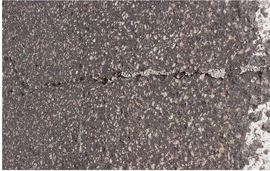
Figure 33. Close-up View of Vibratory Scraping on the Roadway
