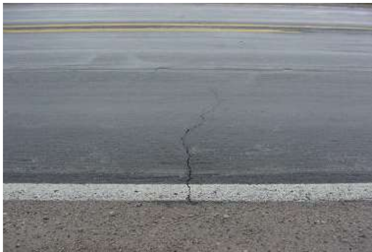
Figure 40. Close-up View of Some Scraping of the Roadway Surface and Overall Poor Condition of the Roadway
