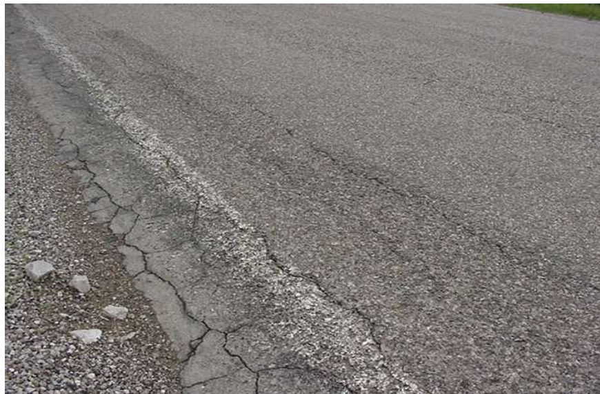
Figure 43. Close-up View of Cracking Along Edge
