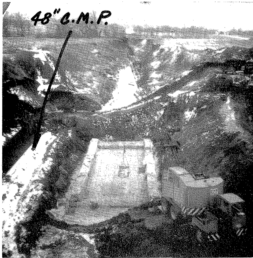
Figure 2 - Placement of Gabions for Stilling Basin
