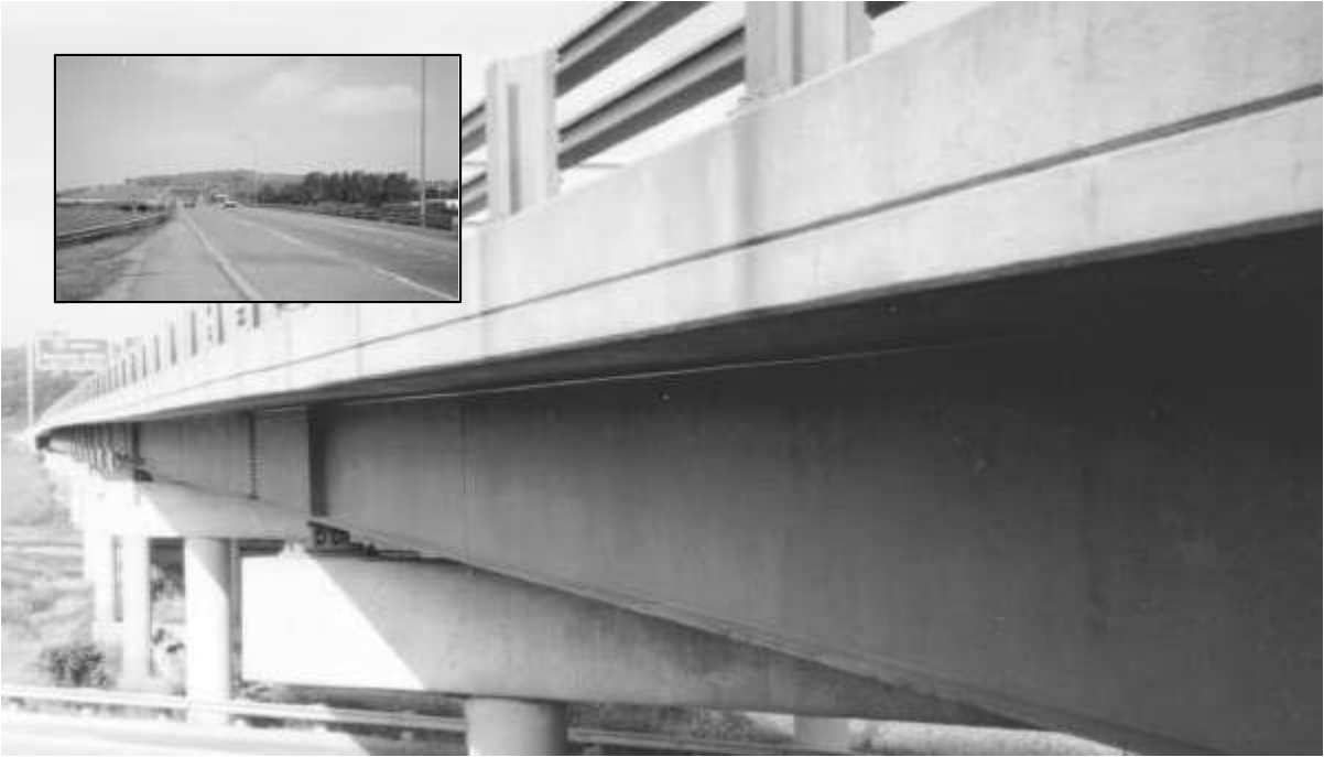
(a) Overview and roadway
