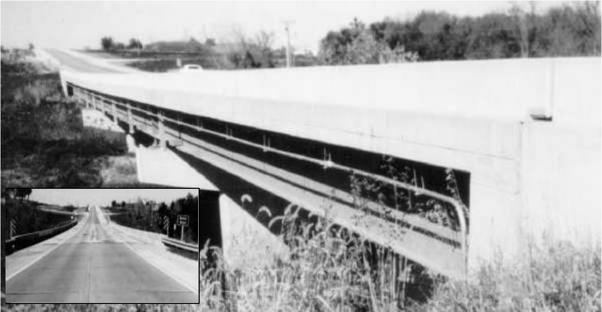
(a) Overview and roadway
