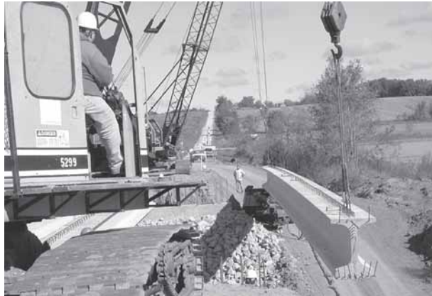
Placing the third bridge beam
