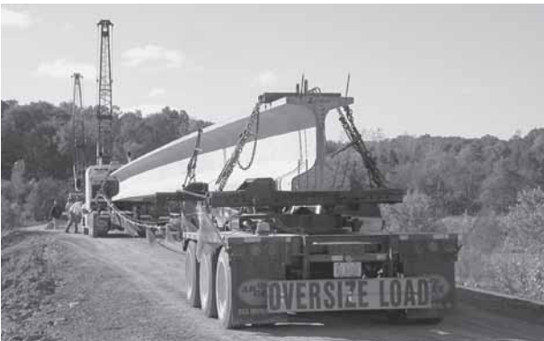
One of the beams, as delivered to the site from Winnipeg
