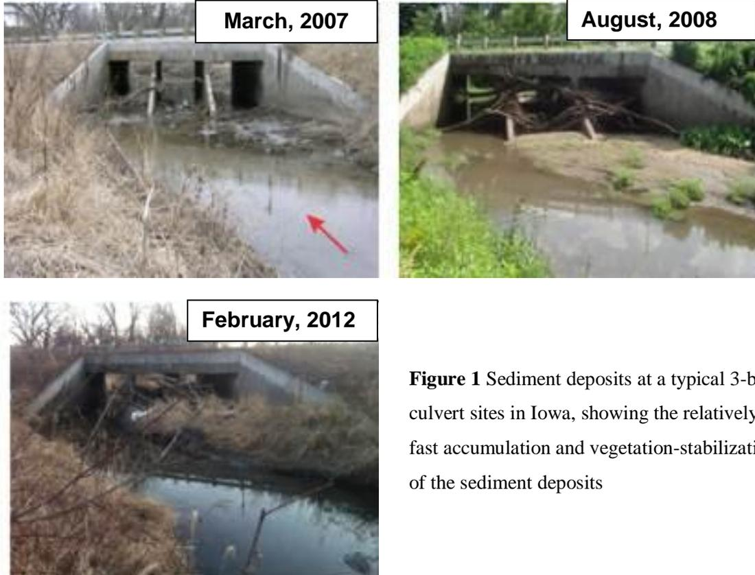
**Figure 1** Sediment deposits at a typical 3-box culvert sites in Iowa, showing the relatively fast accumulation and vegetation-stabilization of the sediment deposits
