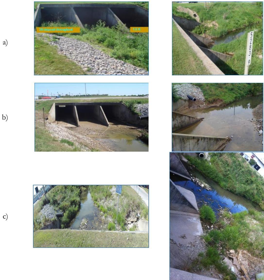
**Figure 13** The culvert site under monitoring on Hwy 1, Iowa City: a) before cleanup (September 15, 2010); b) the culvert right after the September 15, 2010 cleanup; c) the status of the culvert after two years of operation (August 29, 2012)
