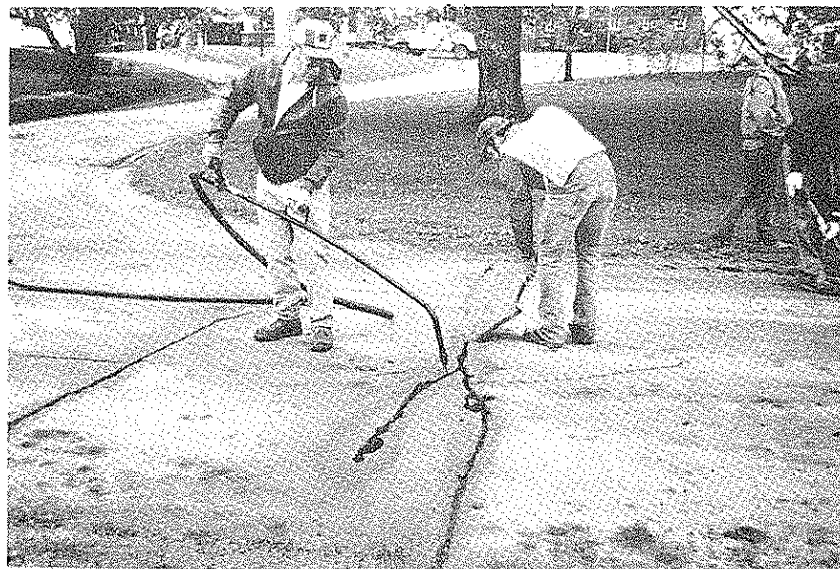
Figure 6 Crack Filling With Emulsion From A Wand
