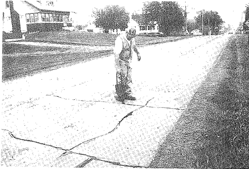
Figure 7 Crack Filling With Emulsion From A Pour Pot
