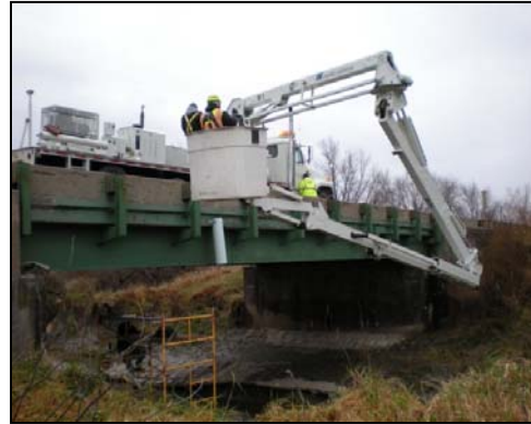
Figure 3 Snooper truck used to access the superstructure of the field bridge during controlled vibration tests
