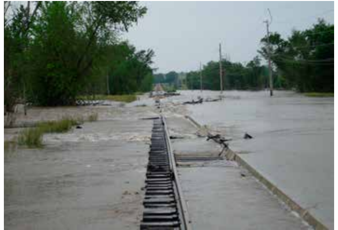
Flooding on the Iowa River in 2008 caused significant damage to the CRANDIC rail line near Amana and significant shipping delays for the railroad's customers.
