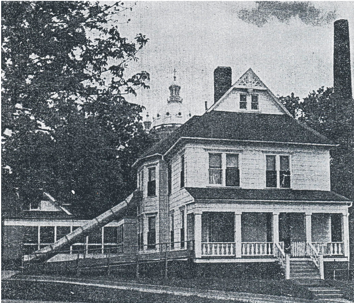
This frame house on Des Moines Street has been a private home, a governor's residence, headquarters for the State Department of Health and Vocational Education Training Center—its present role. Ramps and a fire escape chute on the left side of the building were installed because handicapped persons receive training there. The tip of the Capitol dome rises above the trees.
