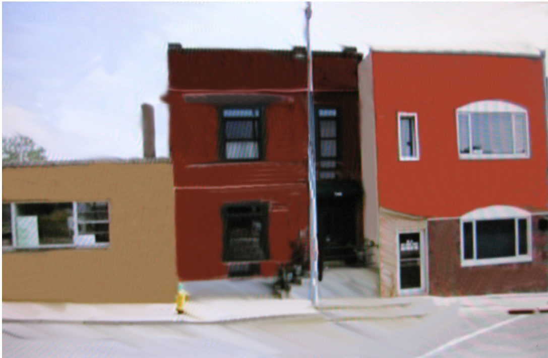
At the base of the West Capitol Terrace stand two 1890s row houses and a 1950s office building. The office building at the far left was a medical building in the 1950s. The building at the far right once housed the medical office of Dr. James Taggart Priestly.
