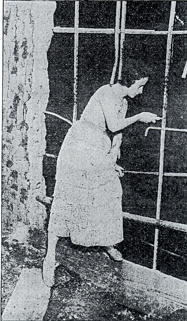
How spooky it looks, this tunnel way below the surface of the ground. Dolores Madole of Dows is exploring the abandoned concrete passage underneath the state house. Part of it is to be used to carry steam to the remodeled Amos Hiatt school at East Twelfth st. and Court ave., which is to house state offices after Sept. 1.
