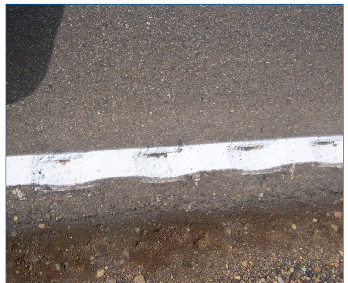
Completed edge-line rumble stripe on a rural HMA highway in Iowa
