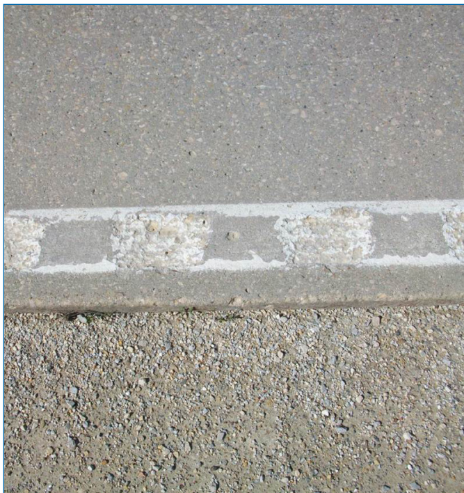
Sample wear on PCC after two winters
