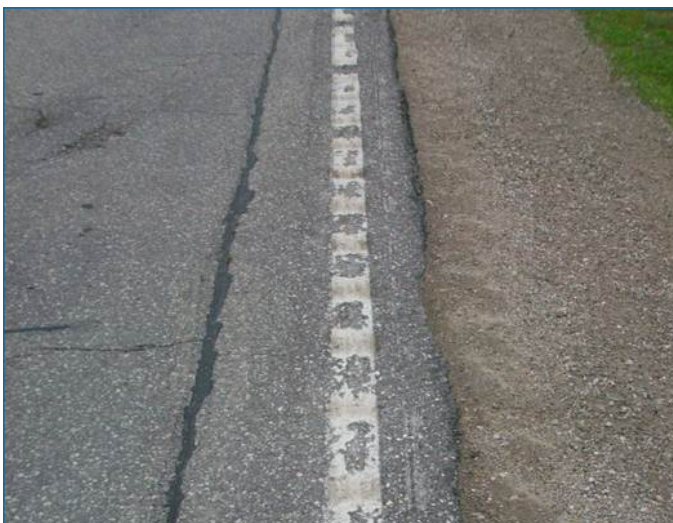
Sample wear on HMA after two winters
