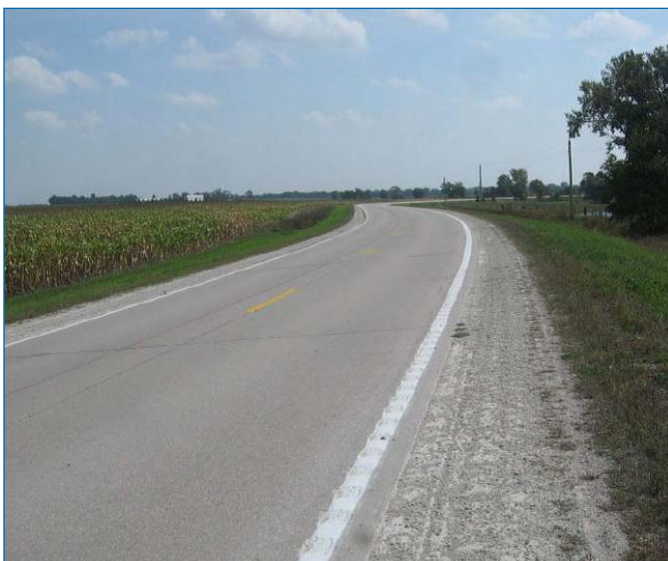
Completed PCC rumble stripe installation in Buchanan County (image: Hawkins, CTRE)
