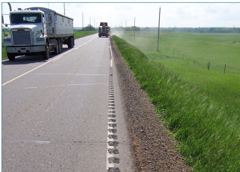
Milling work for edge-line rumble stripes on a rural highway in Iowa
