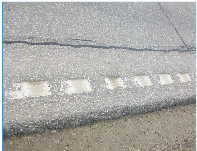
Edge lines still visible in rumble stripe depressions after wear
