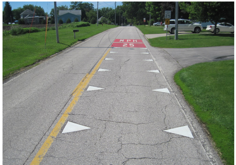
Colored entrance treatment with addition of dragon's teeth for north community entrance to Ossian
