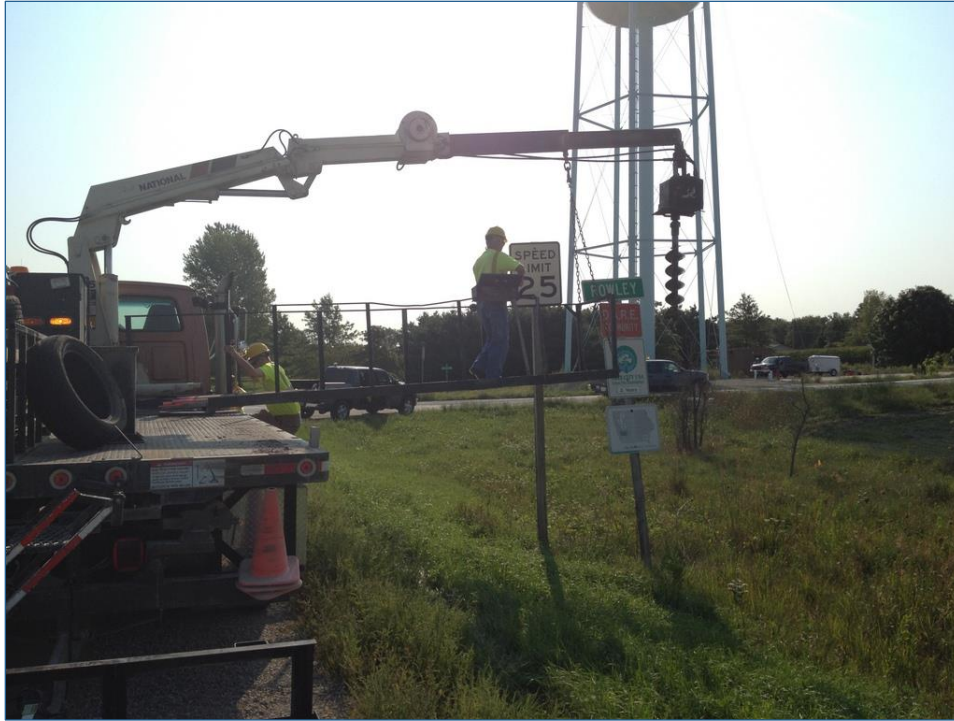
Figure 3-13: Installation of LED speed limit sign
