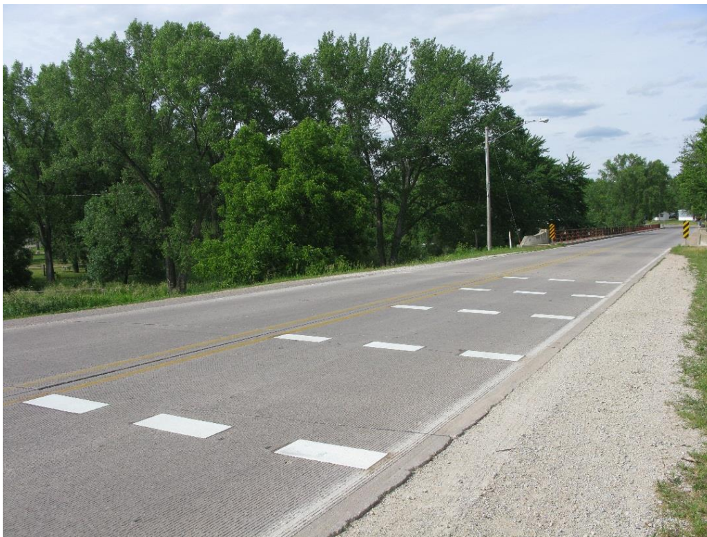
Figure 5-12: Close-up of transverse treatment at south Quasqueton entrance
