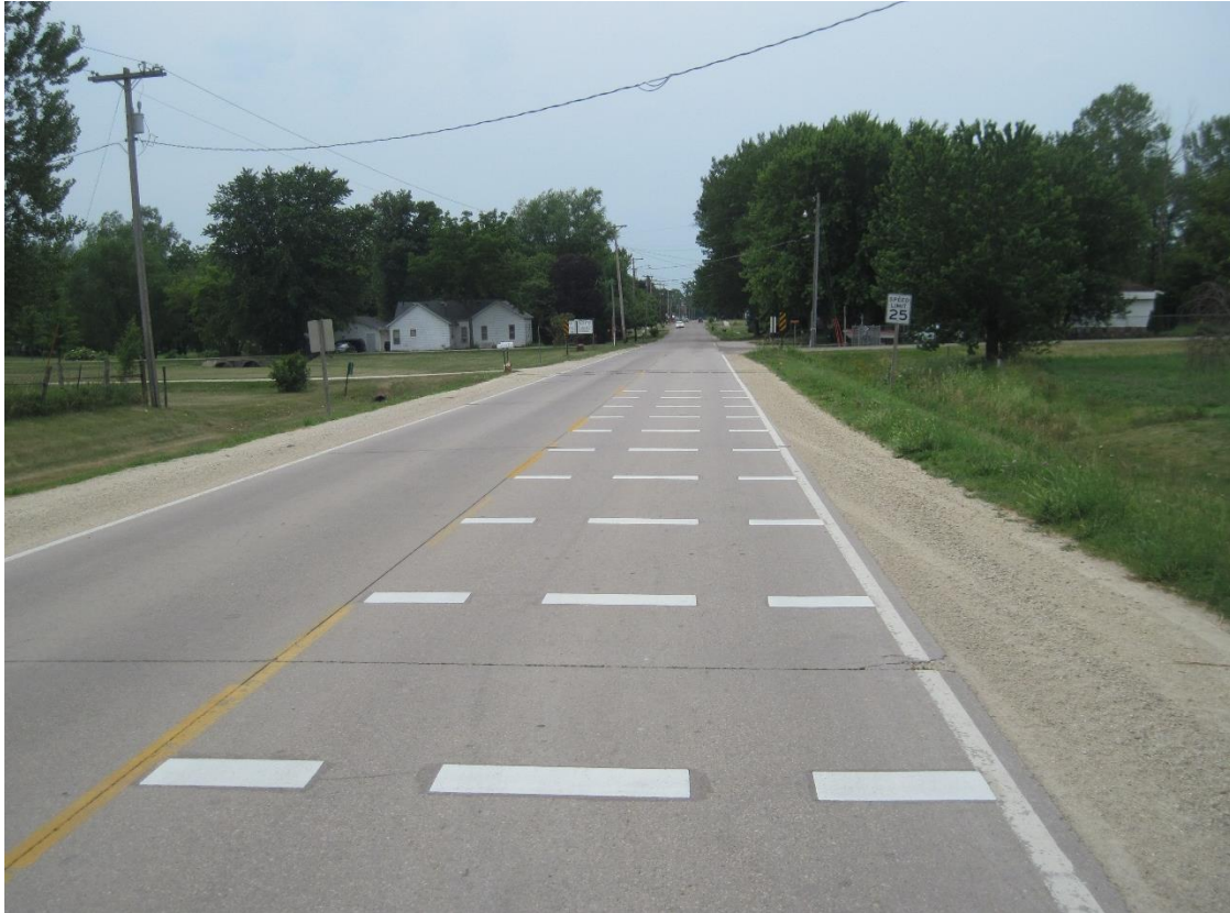
Figure 5-2: Transverse bar treatment at Hazleton east entrance
