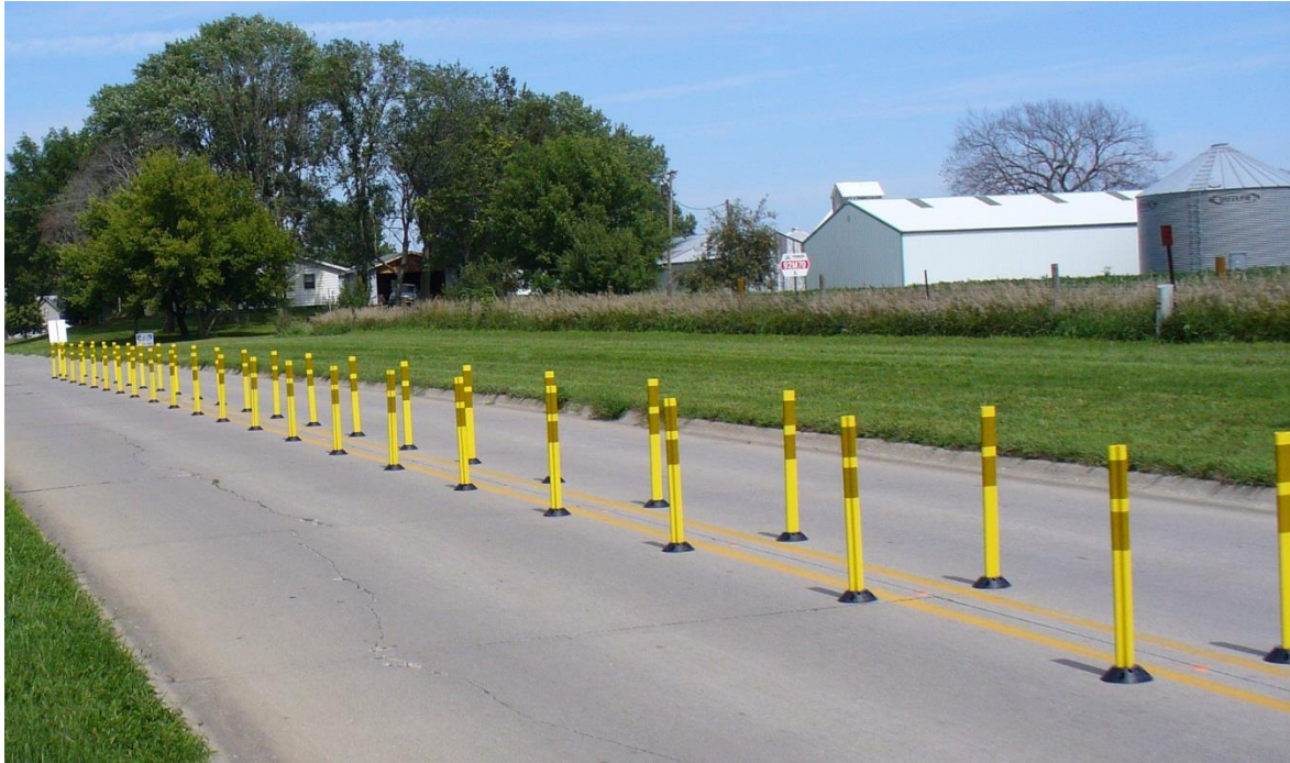
Figure 3-9: Temporary island treatment in Slater, Iowa (Hallmark et al. 2007)
