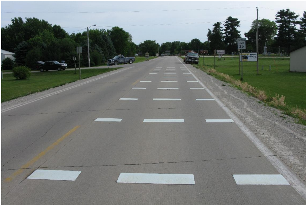
Figure 5-11: Transverse bar treatment for north Quasqueton community entrance
