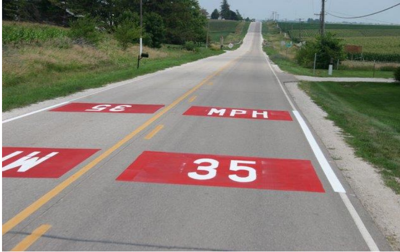
Figure 3-5: European-style traffic-calming treatment used in Dexter, Iowa
