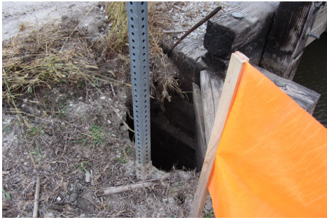
Erosion of abutment backfill
