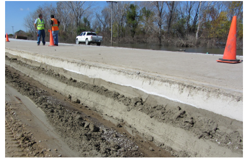
Cement grouting to fill eroded base
