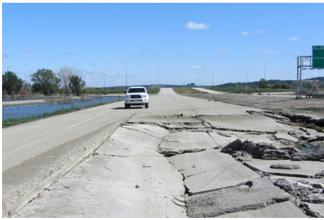
Pavement damage due to erosion
