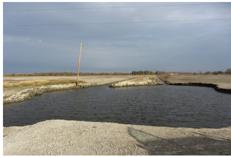
Full breach of roadway embankment
