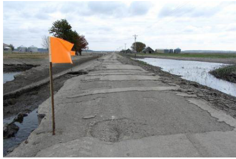
Stripping of chip seal surface
