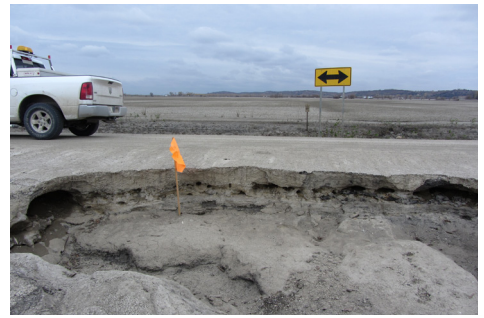
Erosion of granular shoulder
