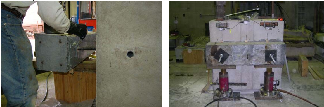
(a) Application of epoxy adhesive (b) Assembled paving notch specimen Figure 4. Photographs of the application of epoxy adhesive and the assembled precast paving notch system.
