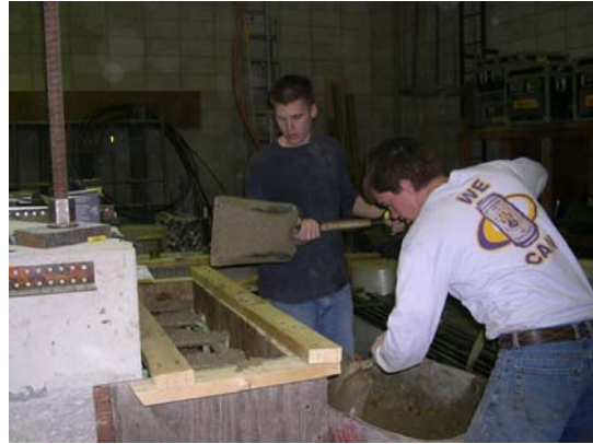
(b) Concrete placement
