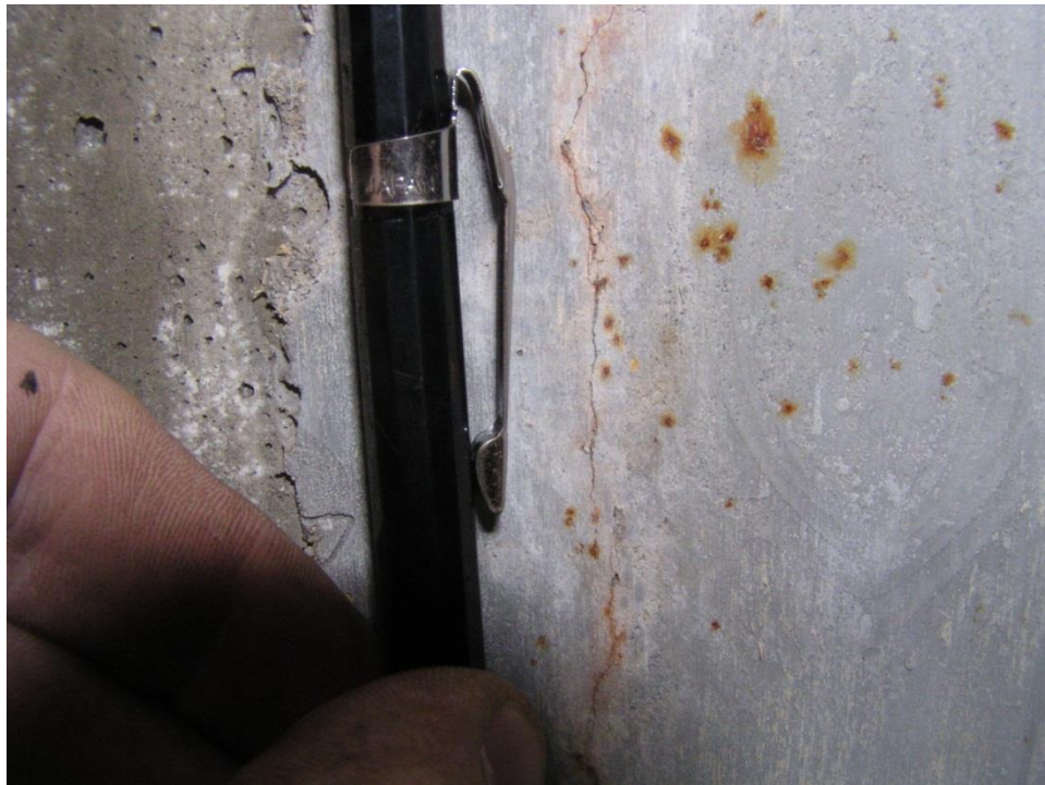
Figure 4.16. Close-up of cracking and efflorescence observed between modules 2 and 3 on bottom of deck
