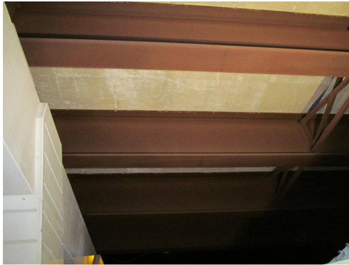
Figure 1. Girders near the intermediate pier; no signs of significant deterioration visible.
