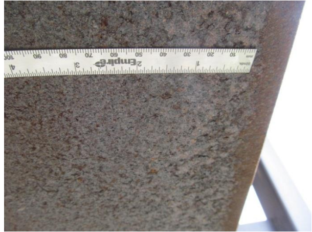
Figure 4. Larger flakes on bottom of fascia bottom flange near downspout by south abutment.
