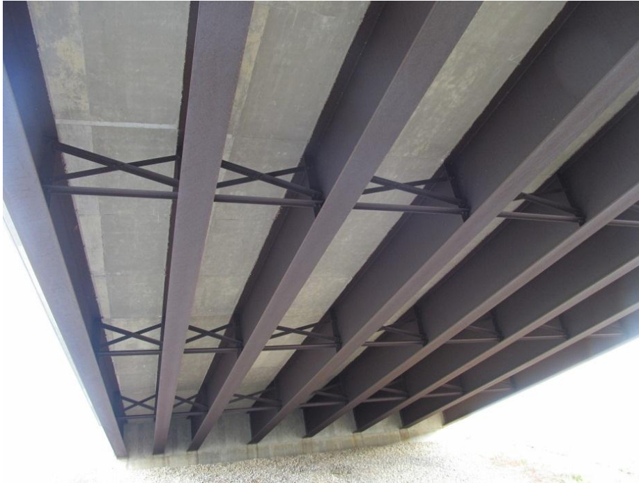
Figure 10. Typical framing for weathering steel bridges in Iowa, note narrow flange width, minimal use of transverse stiffeners, and lack of longitudinal stiffeners and bottom flange lateral bracing.
