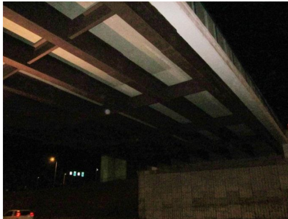
Figure 1. South span over eastbound I-235. Some staining noted on fascia girder and 1st interior girder over the center lane, but not readily visible in this photo.
