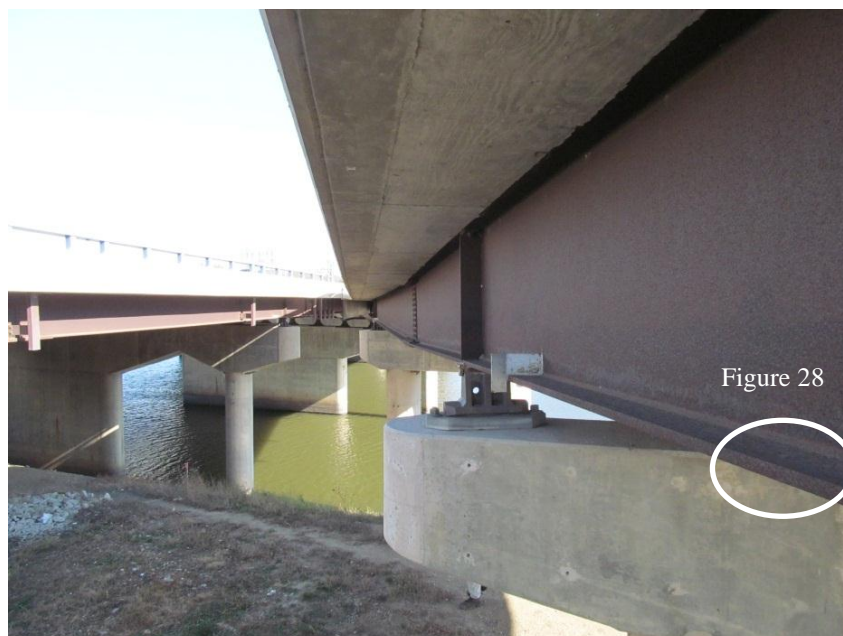
Figure 29. Overall view of I-235 eastbound mainline (left) and on-ramp at 2nd Avenue (right). Note that the portion of the on-ramp fascia girder subjected to salt spray depends on the distance from the mainline structure. As the structures come closer together, the fascia girder is shielded by the deck.
