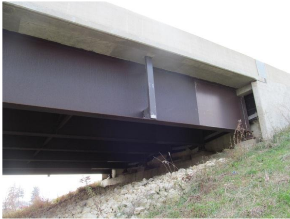
Figure 1. West fascia near south abutment, showing short downspout, painted girder end, and rock apron.
