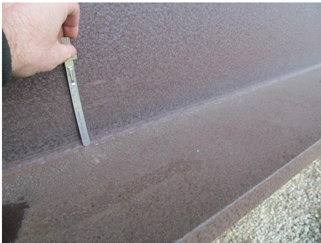
Figure 3. Index 4 and 3 patina on web and top of bottom flange, respectively, near fascia girder tape and chloride tests on 608020.
