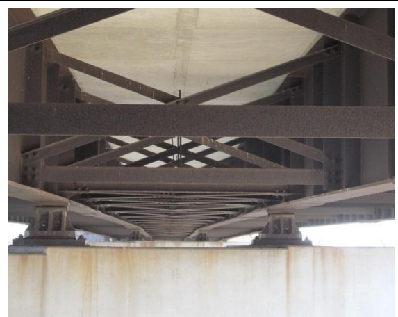
Figure 6. Center bay viewed over top of south pier; note lack of deflector plates and concrete staining.
