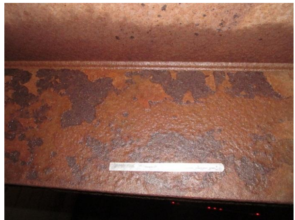
Figure 6. Washing after hand brushing of poultice: Cleaner, but delaminated patina remains.
