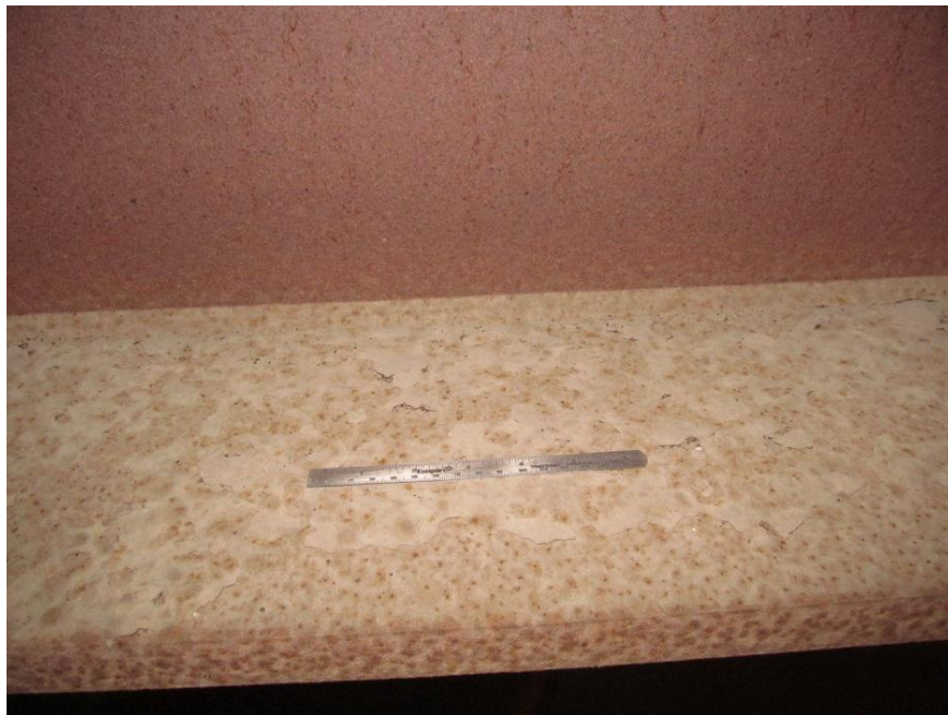
Figure 21. Poultice corrosion on an interior girder flange in downtown Des Moines. This is typical of conditions observed on the tops of many interior horizontal elements. Close examination and testing confirms this chalky film is primarily a mixture of dirt and salts.
