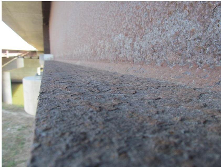
Figure 28. Fascia girder of I-235 eastbound on-ramp at 2nd Avenue. Note transition from Category 3 patina at mid-height of the web to Category 2 at the top of the bottom flange in areas subjected to direct salt spray from the I-235 mainline.
