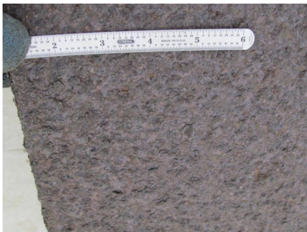
Figure 5. Heavy flaking of bottom of flange in traffic span, typically Index = 2 or worse.
