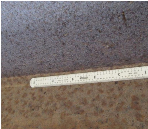
Figure 3. Interior surfaces near east abutment with less deterioration than areas over traffic.
