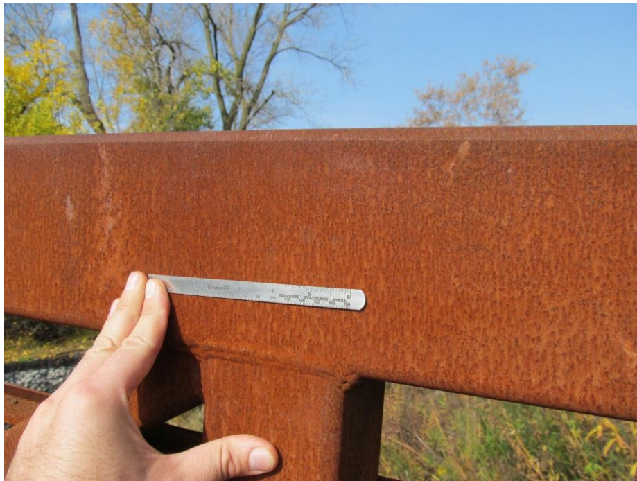
Figure 5. Developing patina on pedestrian bridge in a suburban Illinois park. Note the adherent, small size of the patina rust particles, and the reddish coloration.
