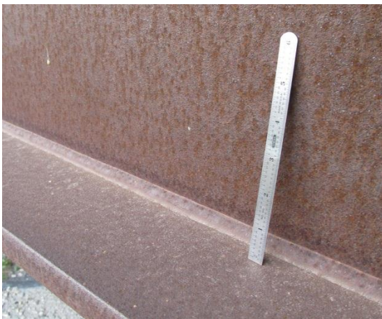
Figure 5. Excellent patina performance on exterior fascia faces after 40 years, typical of rural bridges.
