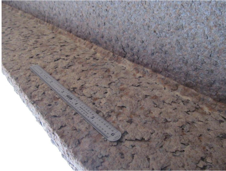
Figure 20. Category 1 patina on top of an interior girder bottom flange; note the large, loose, thick flakes that cover virtually the entire surface. Section loss is not yet apparent in this case.
