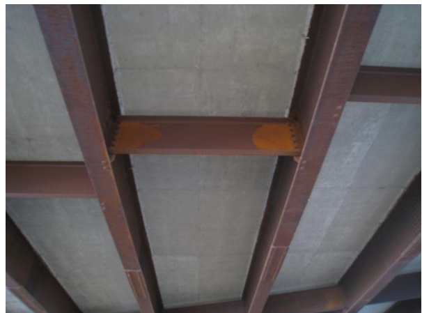
Figure 6. Areas of underdeveloped patina due to spill during construction or mill scale (Index=5).
