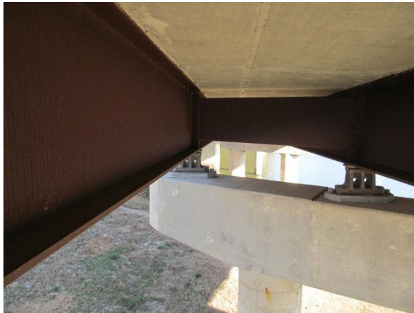
Figure 3. Interior side of entrance ramp north fascia girder demonstrating good patina performance.
