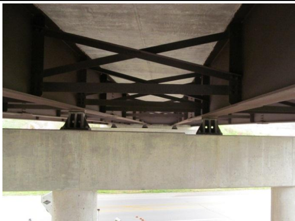
Figure 1. View of south pier looking north; note lack of drainage deflector plates on bottom flanges, typ.
