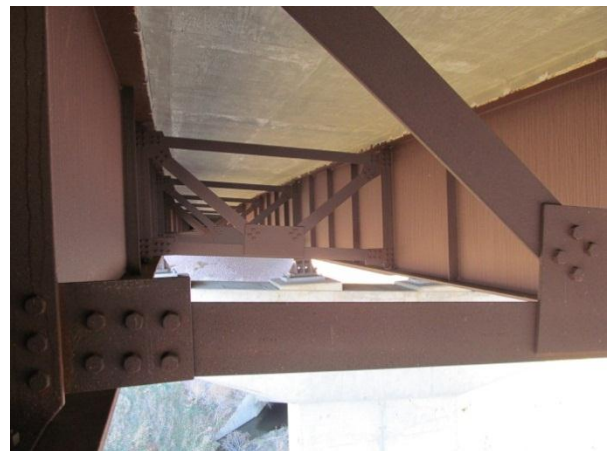
Figure 6. Typical condition of other interior surfaces away from deck cracks typically Index = 3 to 4, with little to no surface chlorides measured.
