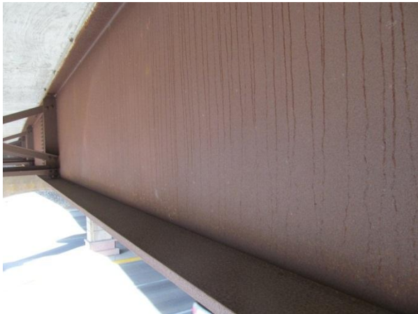
Figure 1. Typical interior girder conditions; good patina performance on web and flange, despite flange poutlice.
