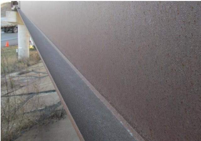
Figure 3. West fascia girder exterior; Index = 3.5 after over 40 years of service.
