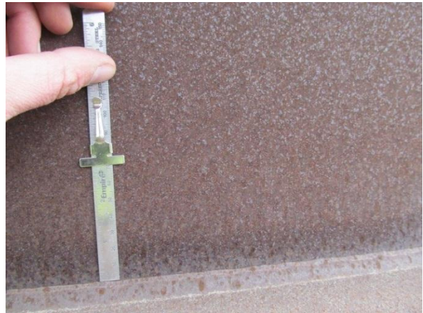
Figure 2. Fascia girder exterior web patina over traffic (Index = 4). Note darker band above weld.
