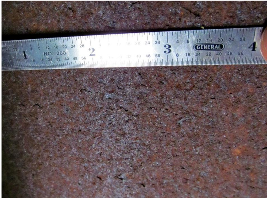
Figure 18. Close-up photo of Category 3 patina on bottom of interior girder web. Texture is less uniform but still generally adherent, with some small loose flakes.
