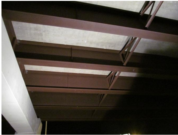
Figure 1. Overall condition of girders and bracing viewed from below, here near pier.
