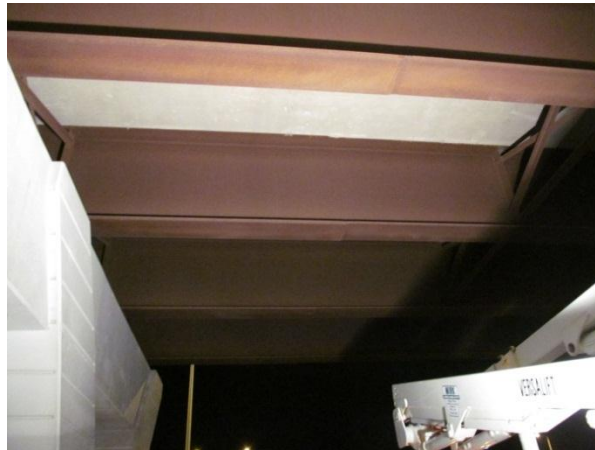
Figure 1. Bottom flanges exhibiting some mild reddish discoloration and possible flaking near pier over eastbound left shoulder.
