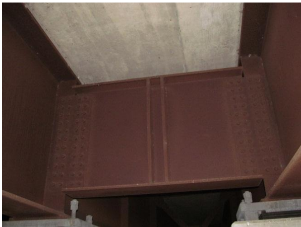
Figure 3. Stiffened I-beam diaphragm at pier.
