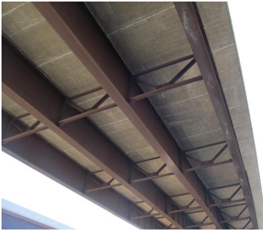
Figure 1. Typical middle bay of southbound bridge; note regular cracking with efflorescence and heavy salt staining on west fascia girder bottom flange.
