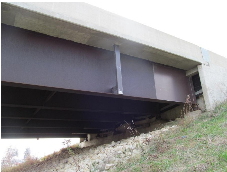
Figure 15. Typical detailing for weathering steel bridges in Iowa, note the painted ends of the girder.
