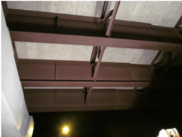
Figure 1. East half of bridge girders near pier; generally good patina condition viewed from below.
