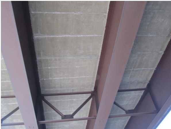
Figure 3. Other girders of southbound bridge show little change in patina condition beneath cracks.
