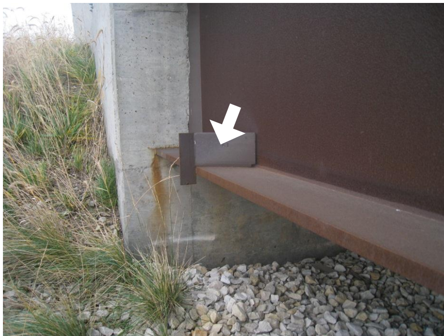
Figure 13. Typical detailing for weathering steel bridges in Iowa, note the water diversion plate (arrow), the painted ends of the girder, and the use of integral abutments.
