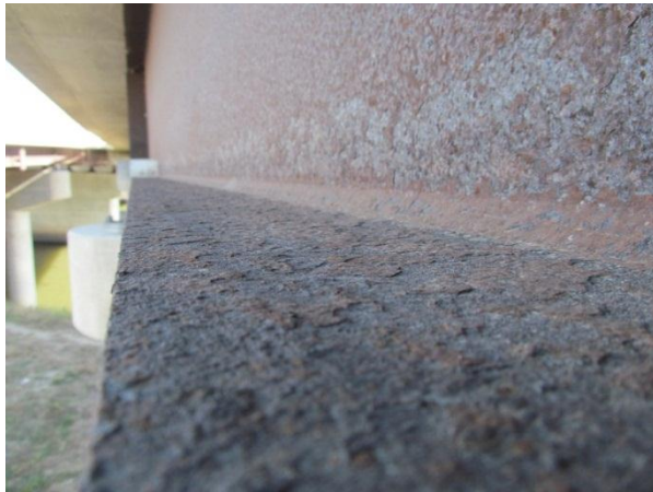
Figure 1. Delamination of top of exterior bottom flange and web of north fascia girder on I-235 eastbound entrance ramp.
