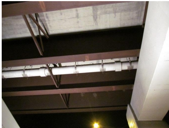
Figure 2. Rectangular, reddish stains on bottom flanges. Also note grayish staining on interior web of fascia girder beyond. Such stains occasionally noticed throughout Field Selection 7.
