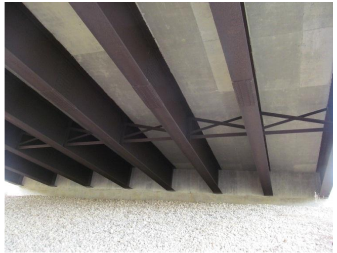
Figure 2. Typical conditions underneath interior of both bridges. Index = 3.5 to 3 on bottom flanges. Sound deck prevents water infiltration from above.
