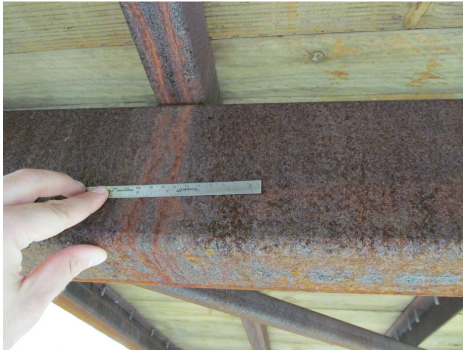
Figure 4. Apparent nonprotective patina on the floor beams and bottom chords of this 10 month old wood-decked pedestrian bridge.
