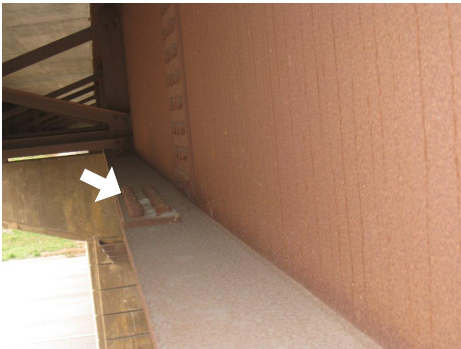
Figure 11. Typical detailing for weathering steel bridges in Iowa, note the narrow flange splice plate that prevents ponding water at the leading edge.
