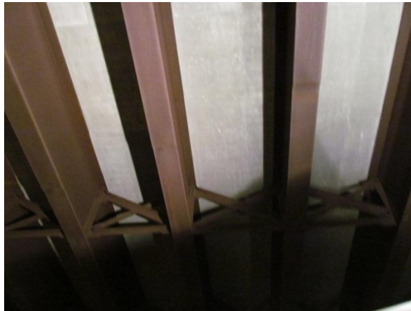
Figure 2. Uniform, dark patina performing well near mid-span.
