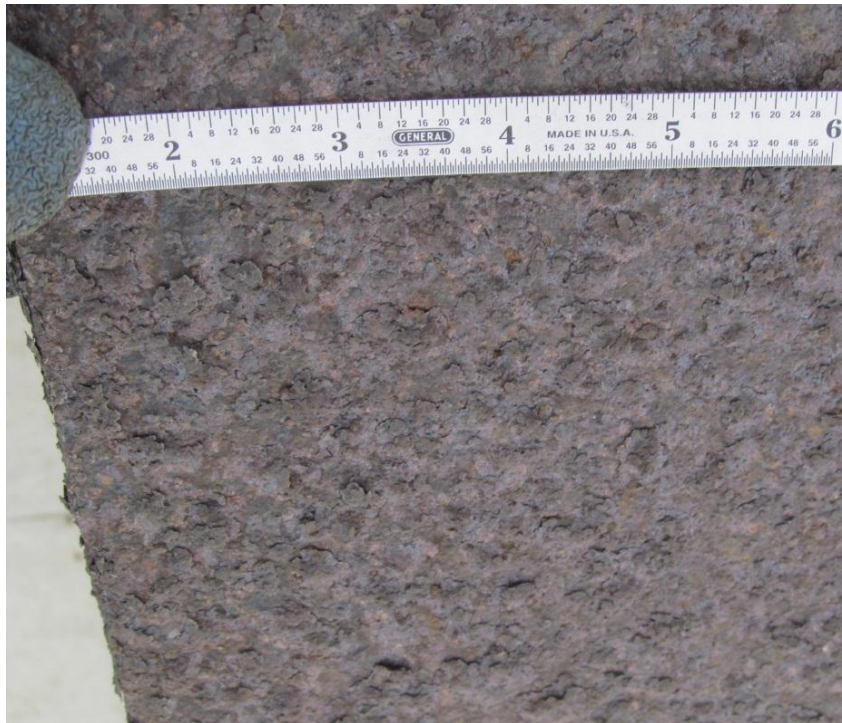
Figure 19. Close-up photo of typical Category 2 patina on the underside of an interior girder bottom flange. Medium size flakes are easily peeled away with a fingernail.
