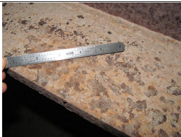
Figure 4. Delamination of interior girder bottom flange with heavy poultice subjected to light scraping.
