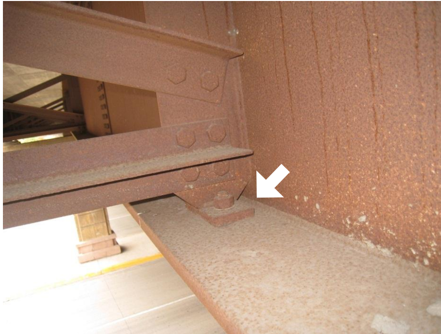
Figure 12. Typical detailing for weathering steel bridges in Iowa, note the coped stiffener that allows water to pass.
