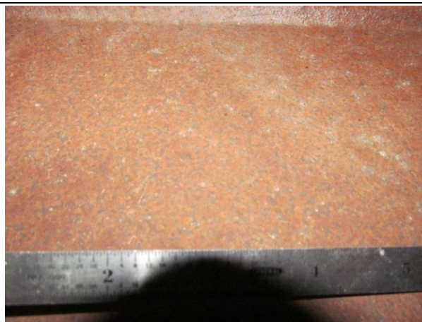
Figure 6. Washed area of top of flange patina after fully dried; adherent, well-behaved beneath chalking.
