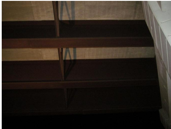
Figure 1. Patina in good condition on all surfaces visible from ground; here near pier.
