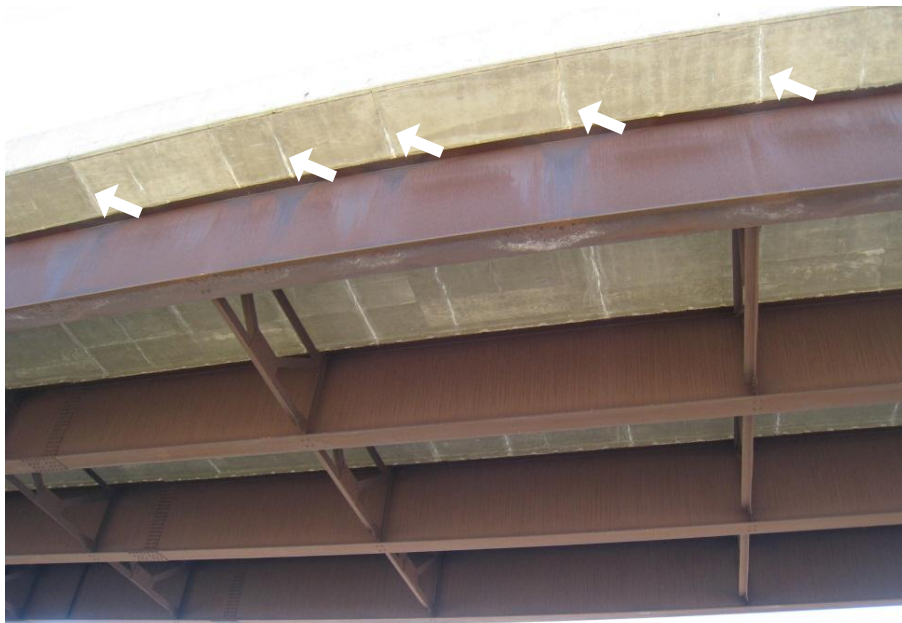
Figure 35. Cracking with efflorescence noted in the concrete deck (arrows) at Structure 9799.5L075, Field Selection 10. Note areas of non-uniform, black weathering steel patina and salt staining on the bottom flange below each crack in the deck.
