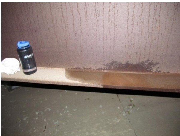
Figure 5. Poultice on east fascia interior side (not flaky). Washed with water and blotted dry.
