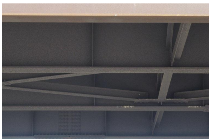
Figure 5. Heavy flaking visible from the ground on interior flanges and webs over traffic lanes; Index = 2.
