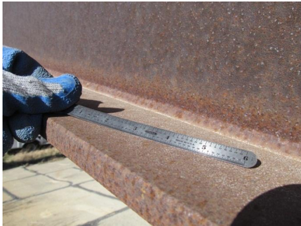
Figure 1. Exterior surfaces over traffic in good condition after more than 40 years.
