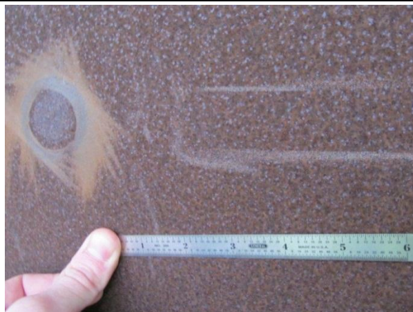
Figure 2. Exterior of east fascia web near south abutment. Index = 4 by tape, chlorides = 0 ppm.
