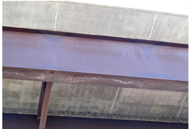
Figure 2. Exterior of west fascia girder on southbound bridge showing localized patina deterioration on all surfaces beneath cracks.
