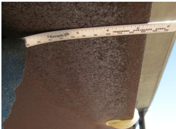
Figure 5. Condition of bottom of flange of east fascia near north abutment considerably better than west fascia (Index = 3).
