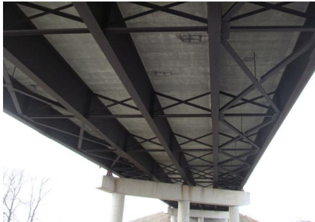
Figure 1. North roadway span showing bracing arrangement and spall locations in the deck.
