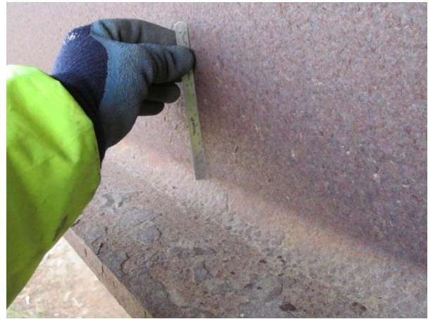
Figure 2. Heavy delamination of fascia bottom flange top (without poultice); also flaky on web.
