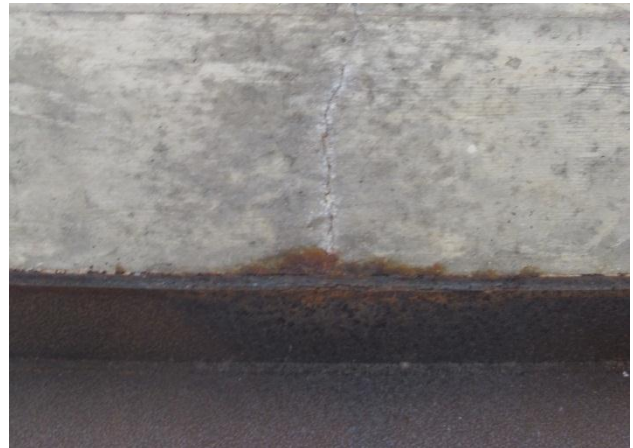
Figure 2. Top flange deterioration beneath concrete deck crack; possibly index rating of 1 on hidden top.
