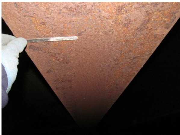
Figure 5. Flaking and small delaminations on bottom of flanges over traffic.
