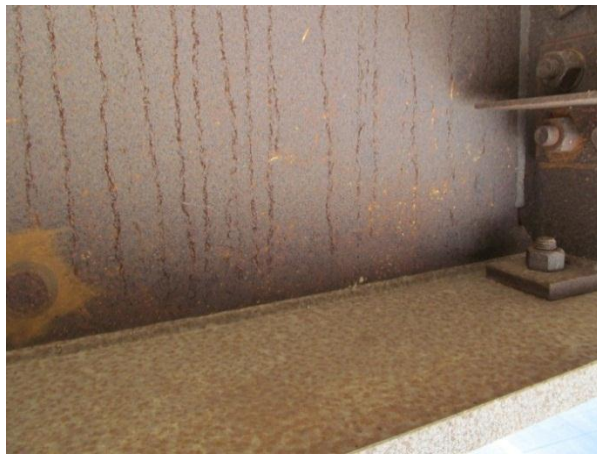
Figure 3. Interior girder over traffic showing poulitice with minimal flaking and reddish web discoloration, possibly due to mill scale.
