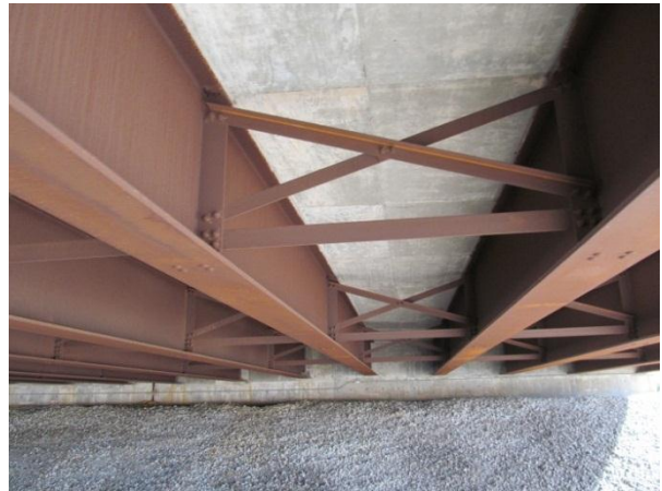
Figure 2. Some discoloration on bottoms of flanges, but only minor flaking. Conditions near abutment similar to those over traffic.
