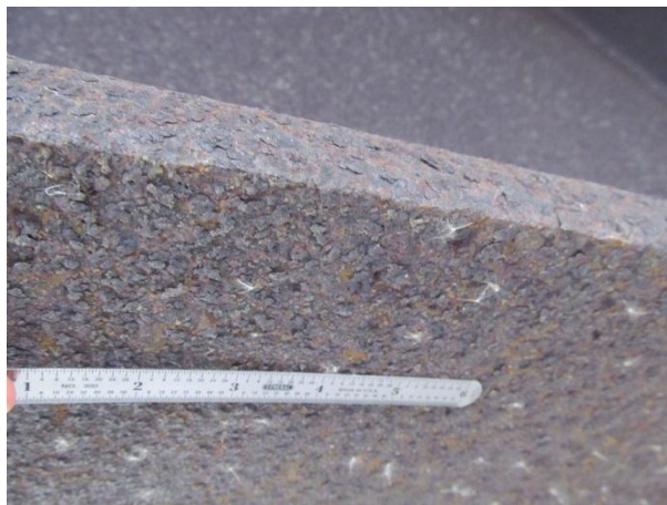
Figure 3. Flakiness on interior bottom flange near south abutment (Index = 2.5). Worse than over traffic on north half of bridge.
