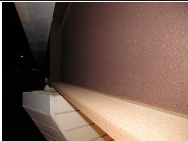
Figure 1. Index = 3.5 to 3 patina on exterior fascia surfaces.
