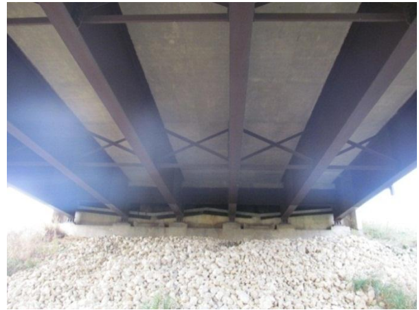
Figure 2. South abutment, showing typical cross-frames and diaphragms detailed to not stain concrete.
