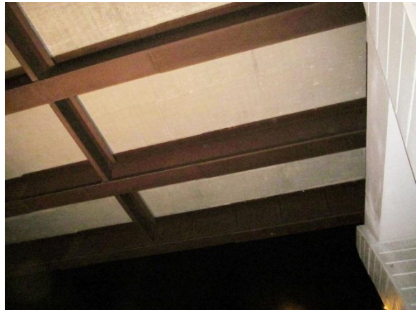
Figure 2. Girders and diaphragms near south pier; appear in good condition from below.
