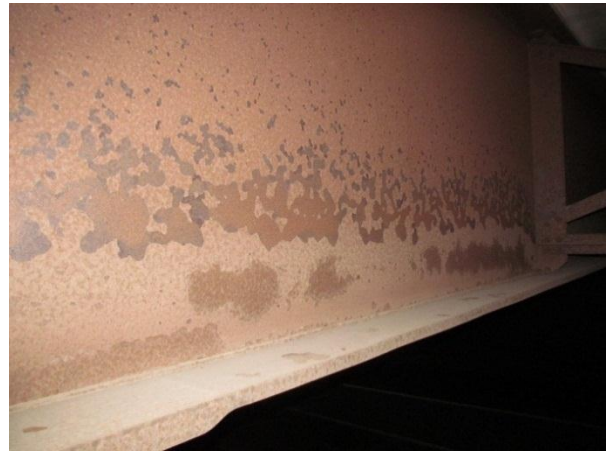
Figure 2. Typical widespread delamination on web above traffic. Lower delaminations appear older, beginning to deteriorate again.
