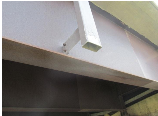
Figure 6. View of downspout; bottom flange corrosion extends away from spout, primarily in direction of girder slope.
