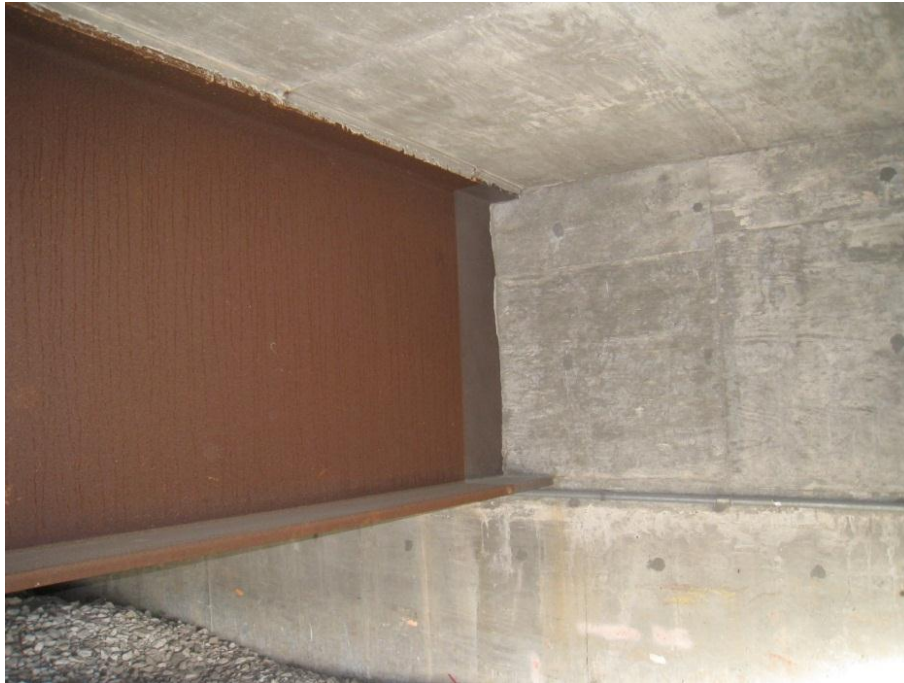
Figure 14. Typical detailing for weathering steel bridges in Iowa, note the use of integral abutments and the painted ends of the girder.
