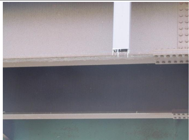
Figure 6. Fascia problems continue over main span.
