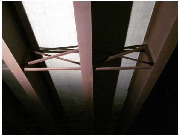
Figure 2. More distinct spots of local discoloration visible near middle of south span.
