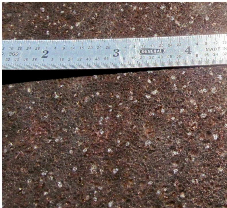
Figure 17. Close-up photo of Category 4 patina commonly observed on exterior web of fascia girder. Surface is textured but tightly adherent, and rust formations are small. No loose flakes are present.
