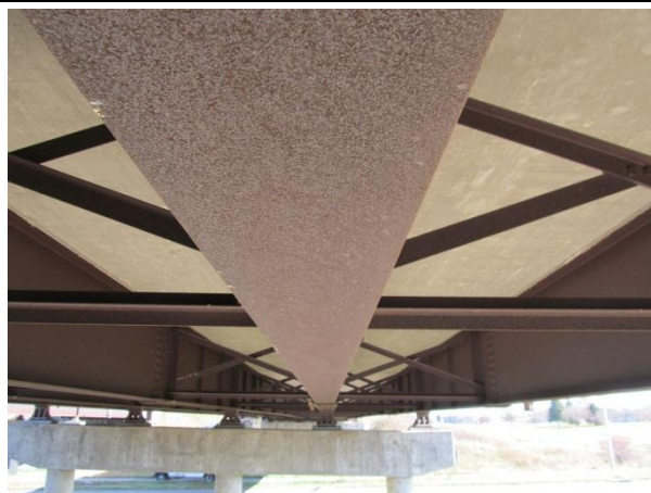
Figure 5. Bottom of flange near west abutment shows less flaking than east side; Index = 3.
