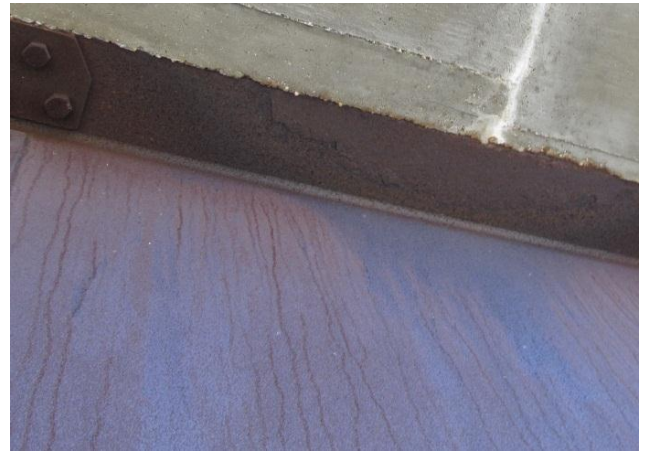
Figure 4. Heavy deterioration/delamination of west fascia girder top flange at crack, possibly Index = 1.
