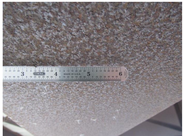
Figure 4. Interior bottom flange condition near north abutment; index here is 3.5. Contrast with Figure 3 from identical location at south end.
