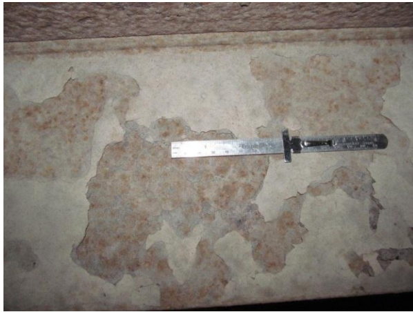
Figure 1. Heavy poultice on interior flange with multiple thin layers of delamination forming.
