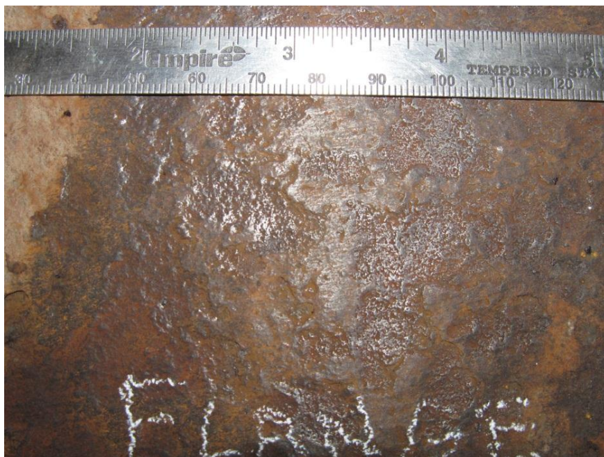
Figure 33. Close-up photo of steel on top surface of girder bottom flange after wire wheel grinding at Field Selection 3; delaminated patina removed down to bare steel with oxide layer remaining in pitted areas.
