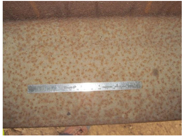
Figure 4. Interior top of bottom fascia flange with light poultice corrosion, but minimal flakiness.
