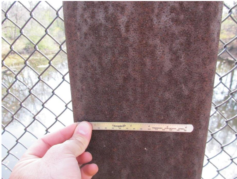
Figure 7. Close-up photo of patina performance on the Des Plaines River pedestrian bridge; patina is dense and adherent, with small constituent rust particles.
