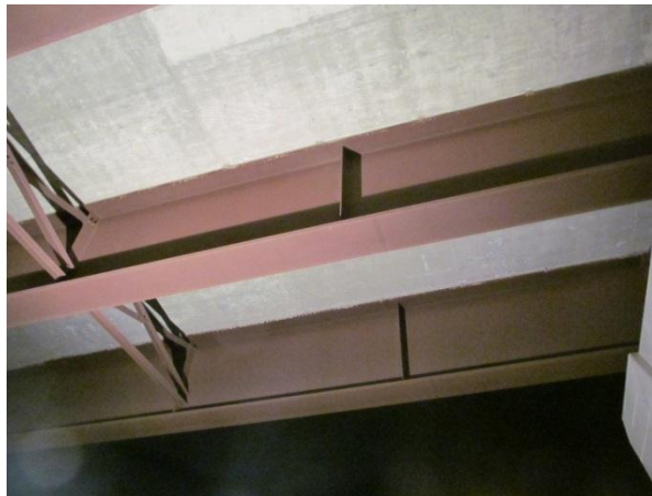
Figure 2. Girders and cross-frames near center pier; no significant deterioration visible from below.
