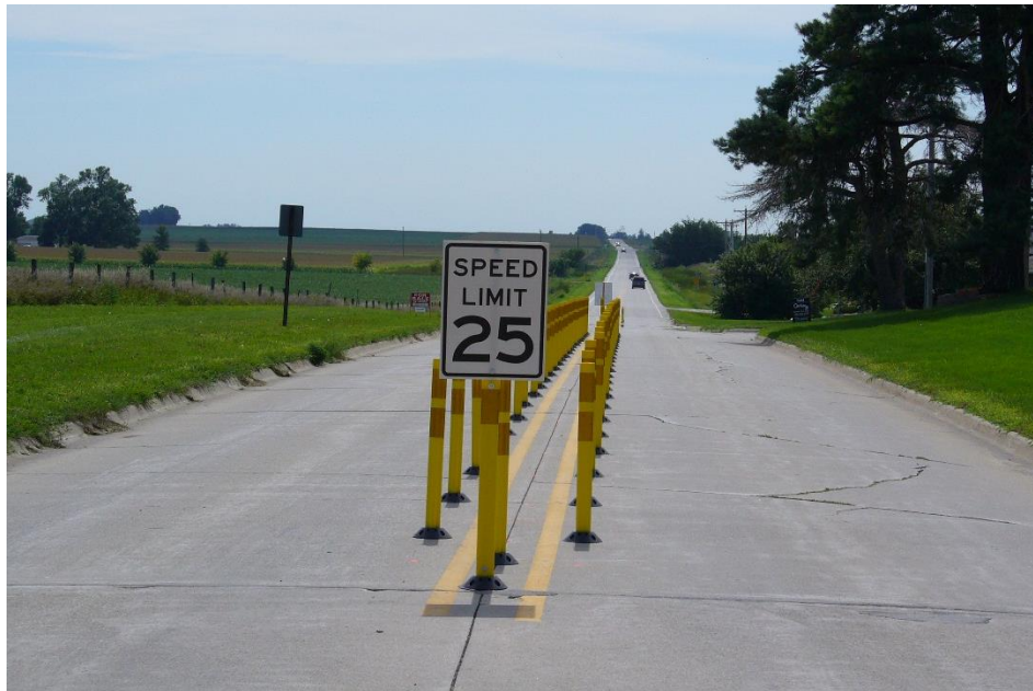
Figure 21: Creation of a center island with channelizers
