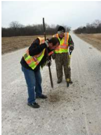
Figure 3. Installation of buried Numetric plate
