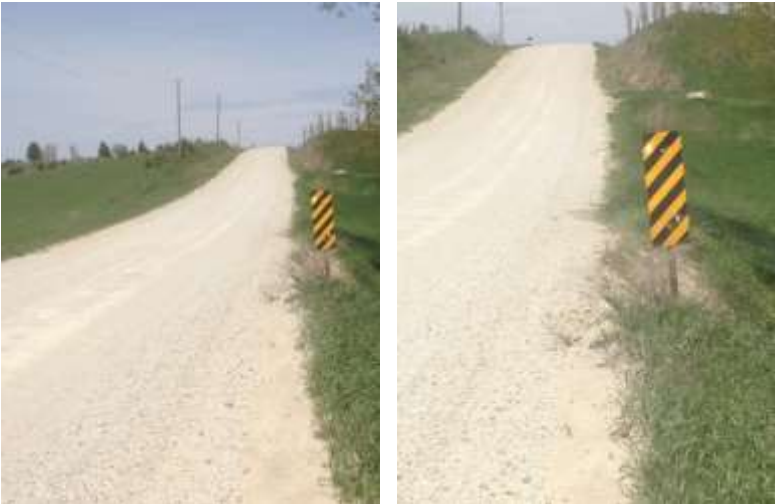
Images of Story County Roadway Signs and Object Markers Installed to Date
