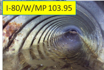
Opened Outlet without Mesh Gate Screen
